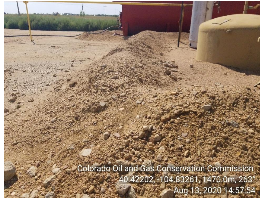
Photo 8: Berm repaired
