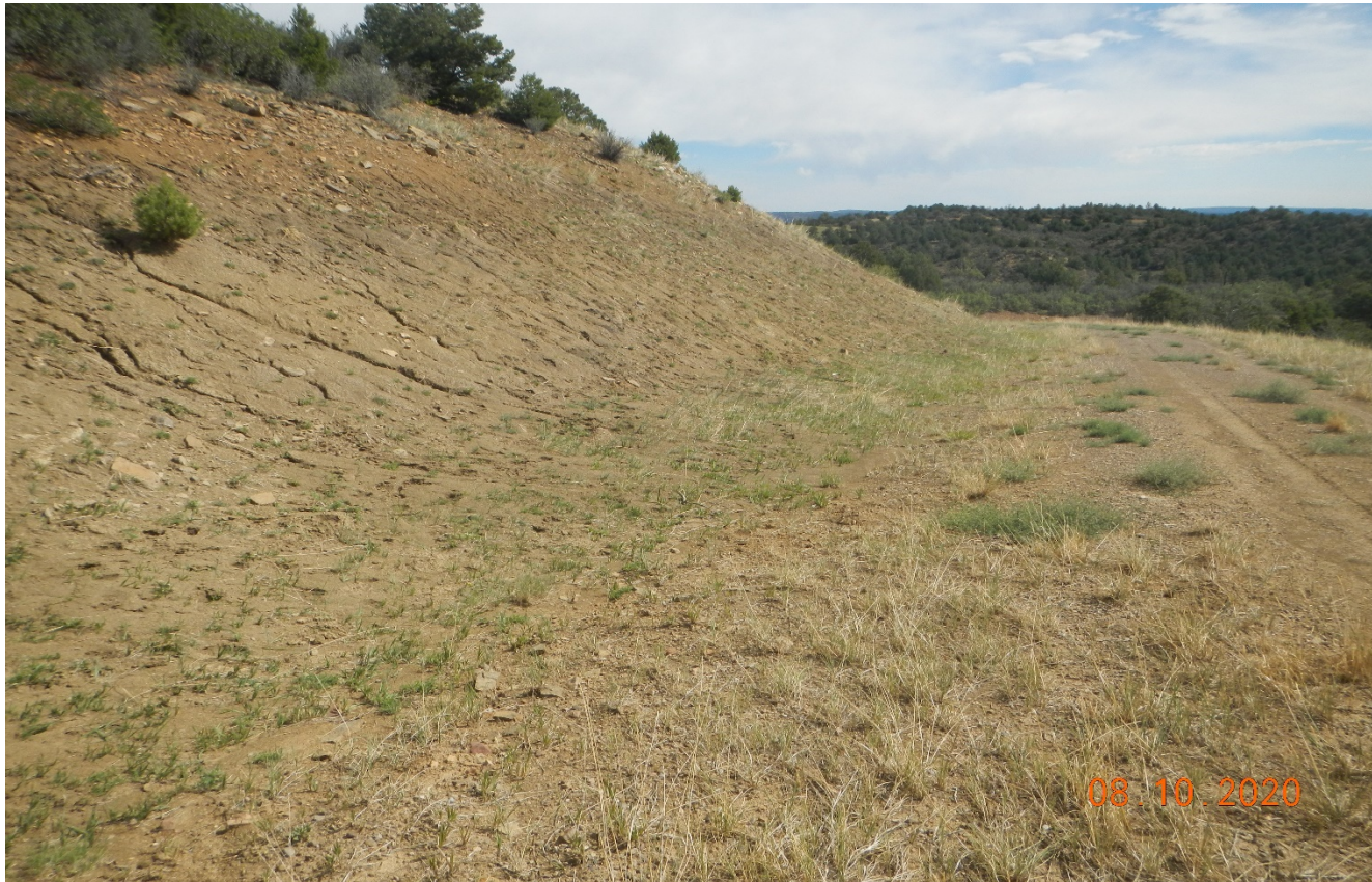
Photo 4. The cut slope along the access road has not established vegetation for long term stabilization. There are signs of erosion along this area.
