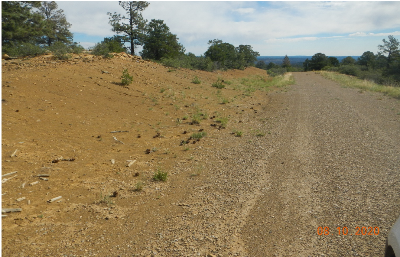
Photo 1. Facing northeast along the access road. The cut slope along the access road has not established vegetation for long term stabilization.
