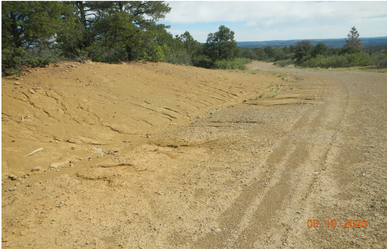
Photo 2. The cut slope along the access road has not established vegetation for long term stabilization. There are signs of erosion along this area.
