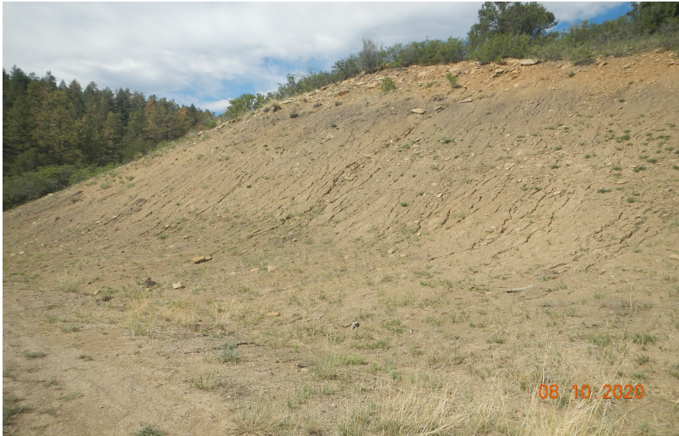
Photo 6. The cut slope along the access road has not established vegetation for long term stabilization. There are signs of erosion along this area.
