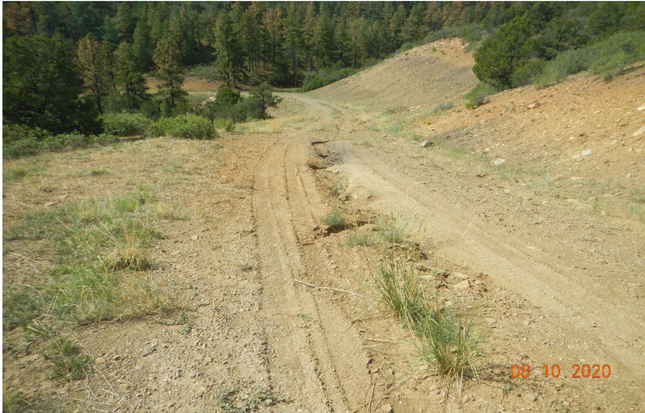
Photo 5. Facing south along the access road. There is an erosion channel along the center of the road ascending down the hillside.
