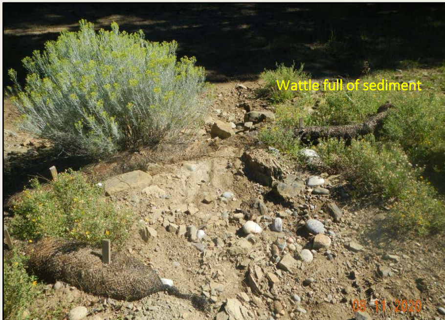
Photos 3/4. View of wattles in the northern and northeastern project area that are full of sediment, displaced, and no longer functioning. Wattles are not adequate BMPs in these areas.
