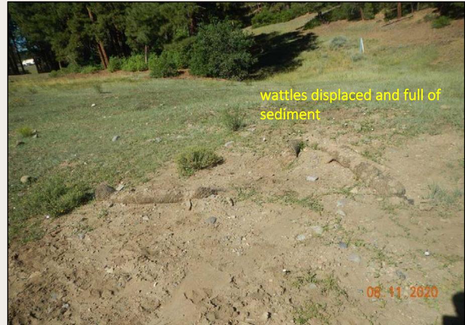
Photos 3/4. View of wattles in the northern and northeastern project area that are full of sediment, displaced, and no longer functioning. Wattles are not adequate BMPs in these areas.
