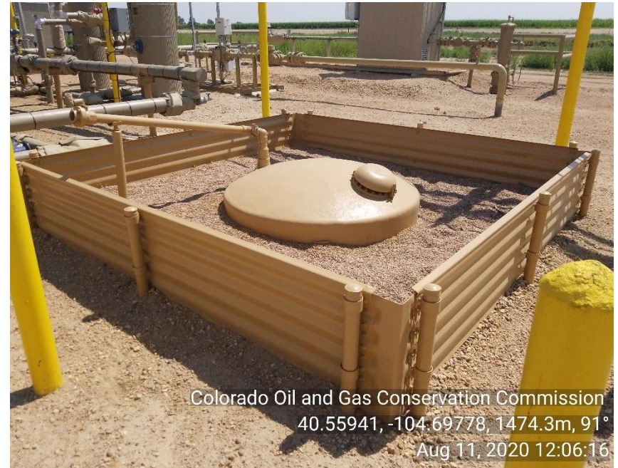
Photo 10: No labeling on tank
