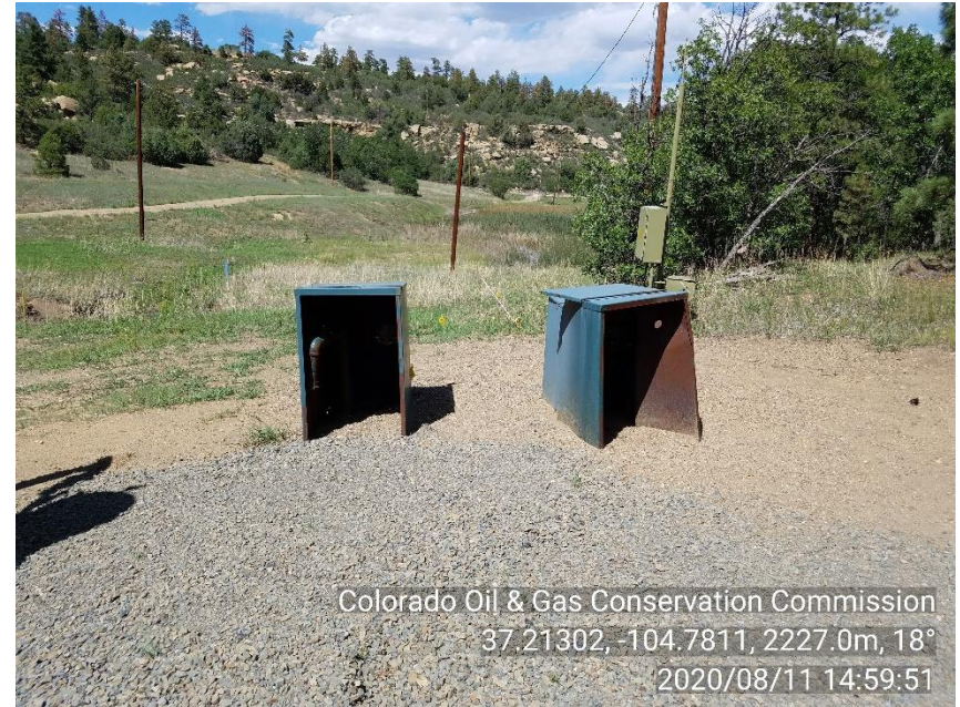
PHOTO 4: UNUSED RISERS UNDER STEEL BOXES NORTHEAST OF METERHOUSE. REMOVE UNUSED RISERS, COMPLY WITH RULE 603.f. CA DATE 11-11-20.
