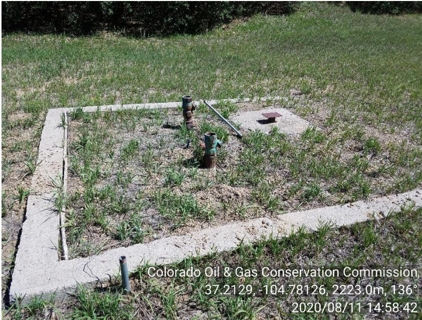
PHOTO 3: UNUSED RISERS JUST SOUTH OF LOCATION. REMOVE UNUSED RISERS, COMPLY WITH RULE 603.f. CA DATE 11-11-20.
