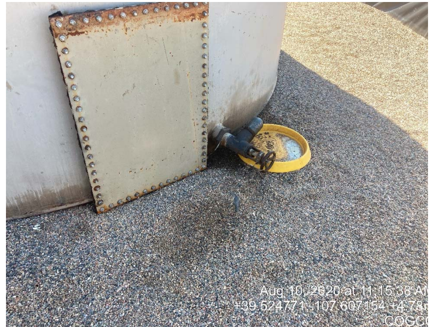
staining under catch bucket
