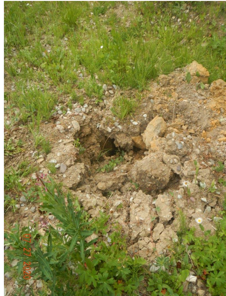
Photo#7: Subsidence that has developed in ditch; position indicated with arrow in Photo#6.
