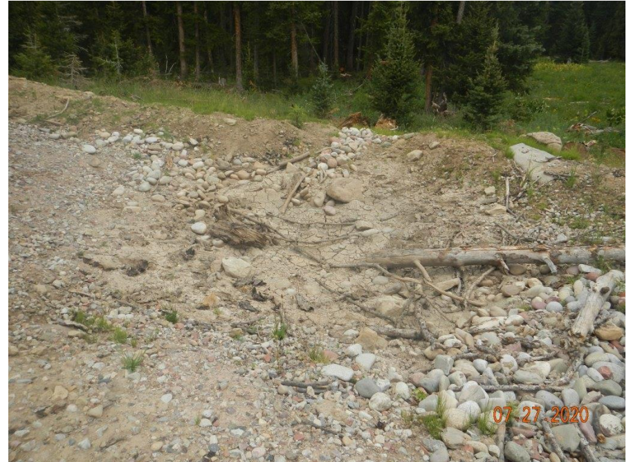
Photo#3: BMP, settling pond 7/27/20; BMP needs maintenance.
