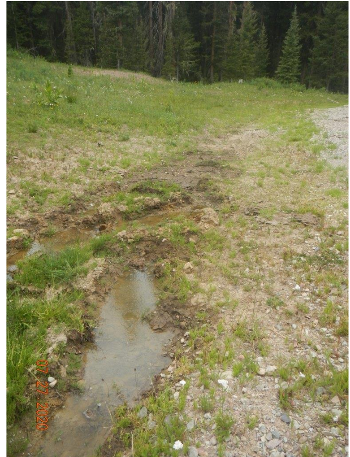
Photo#3: BMP, ditch 7/27/20; BMP needs maintenance.
