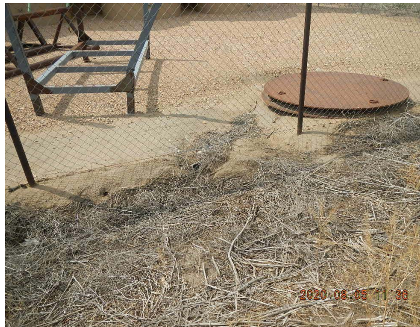
Evidence of sediment leaving the CE&P facility.
