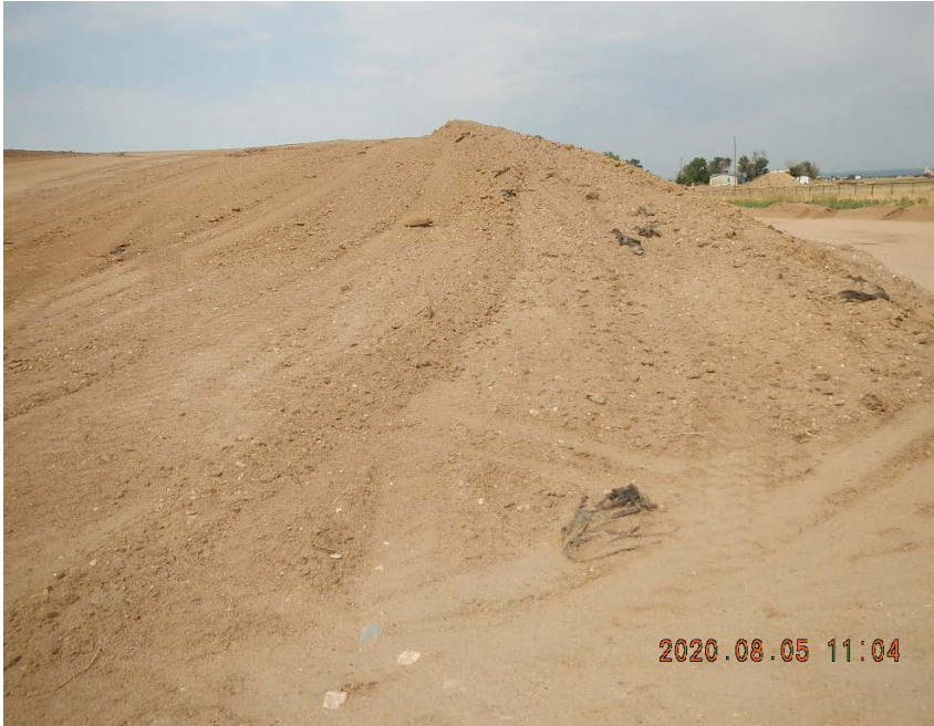
Felt liner incorporated into soil/material mound.
