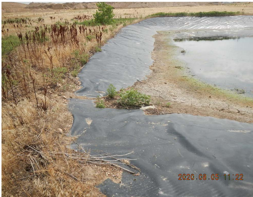
Vegetation and sediment encroachment on liner.
