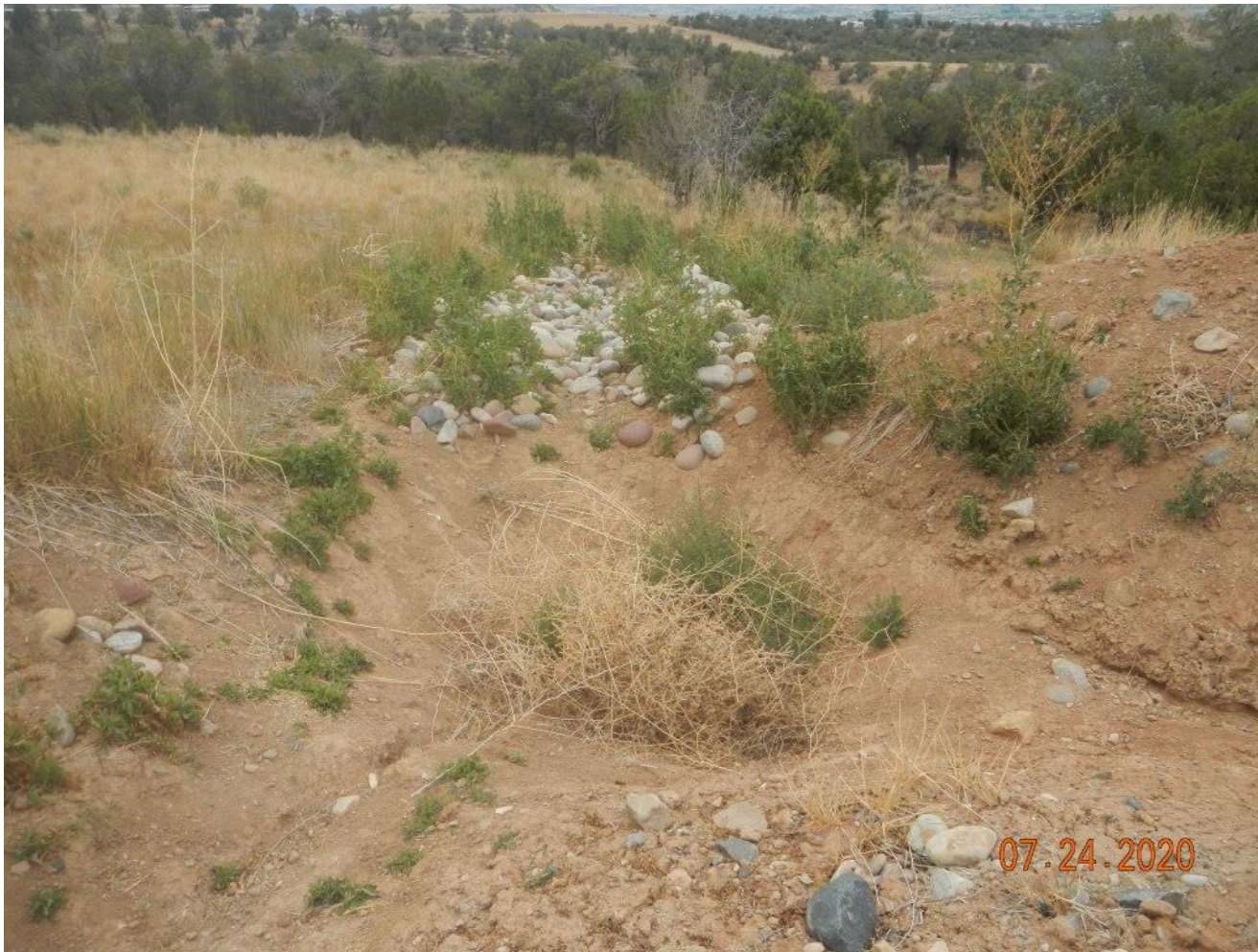
Photo#3: BMP needing maintenance; cleanout of debris weeds.
