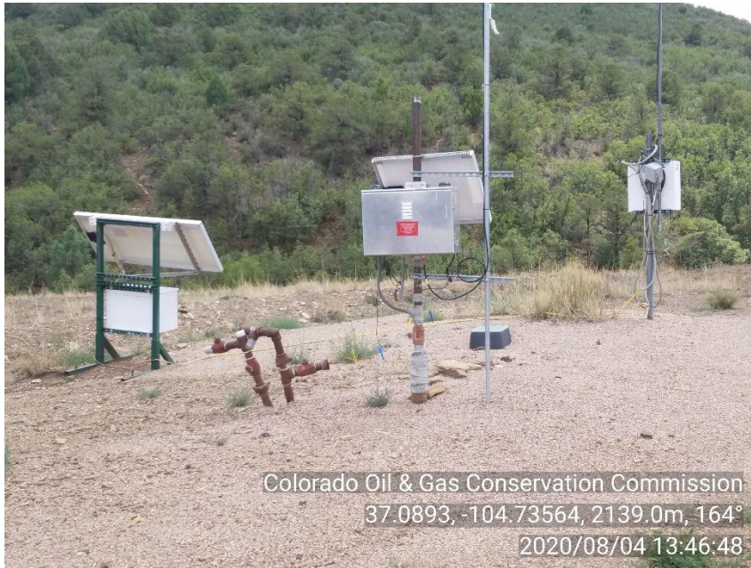
PHOTO 3: UNUSED EQUIPMENT (RISER AND TELEMETRY EQUIPMENT). REMOVE UNUSED EQUIPMENT PER RULE 603.f. CA DATE 11-4-20.
