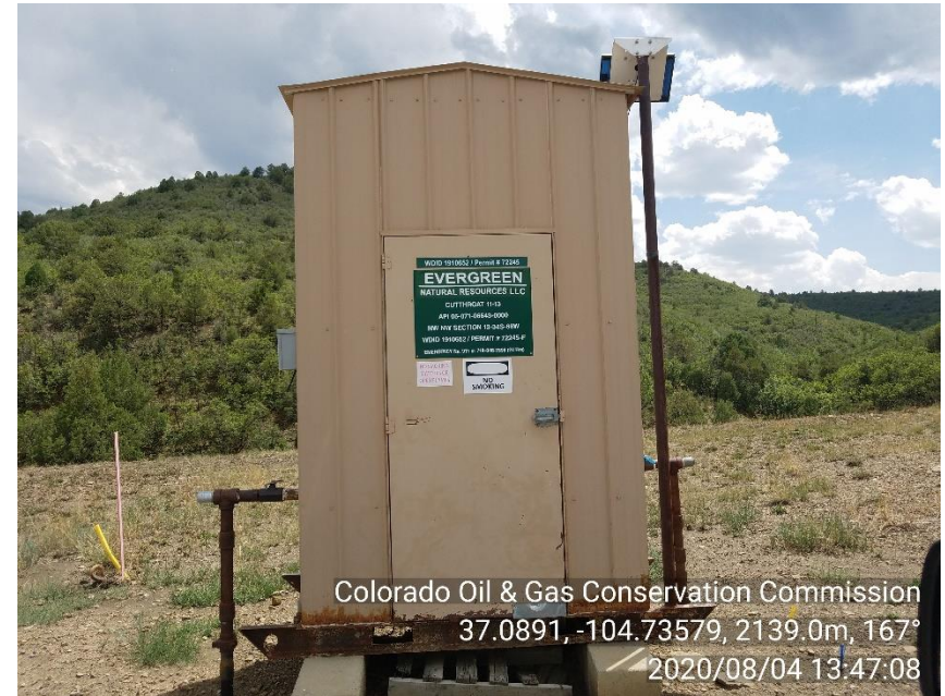
PHOTO 4: UNUSED EQUIPMENT (METER HOUSE). REMOVE UNUSED EQUIPMENT PER RULE 603.f. CA DATE 11-4-20.
