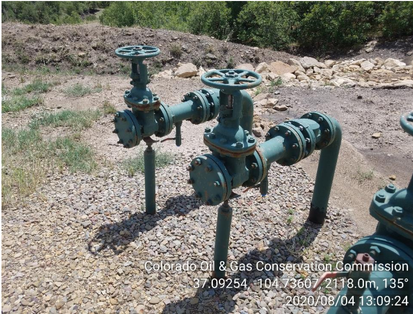
PHOTO 5: UNUSED RISERS (WATER GATHERING LINES). REMOVE OR PUT BACK IN SERVICE. CA DATE 11-4-20.
