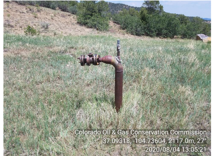
PHOTO 6: UNUSED RISER (GAS GATHERING LINE TO OLD P&A'D WELL) REMOVE UNUSED RISER. CA DATE 11-4-20.
