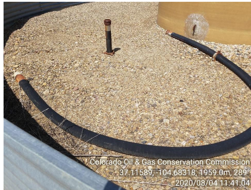
PHOTO 4: UNUSED EQUIPMENT (4" RISER AND 4" HOSE INSIDE SOUTHERN MOST TANK BATTERY CONTAINMENT). REMOVE OR PUT 4" RISER BACK IN USE AND REMOVE UNUSED 4" HOSE. CA DATE 11-4-20.
