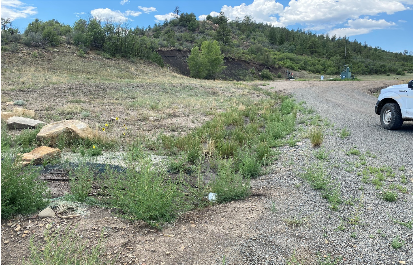
Photo 5. Facing southwest toward the location. This culvert near the location has filled in with sediment.
