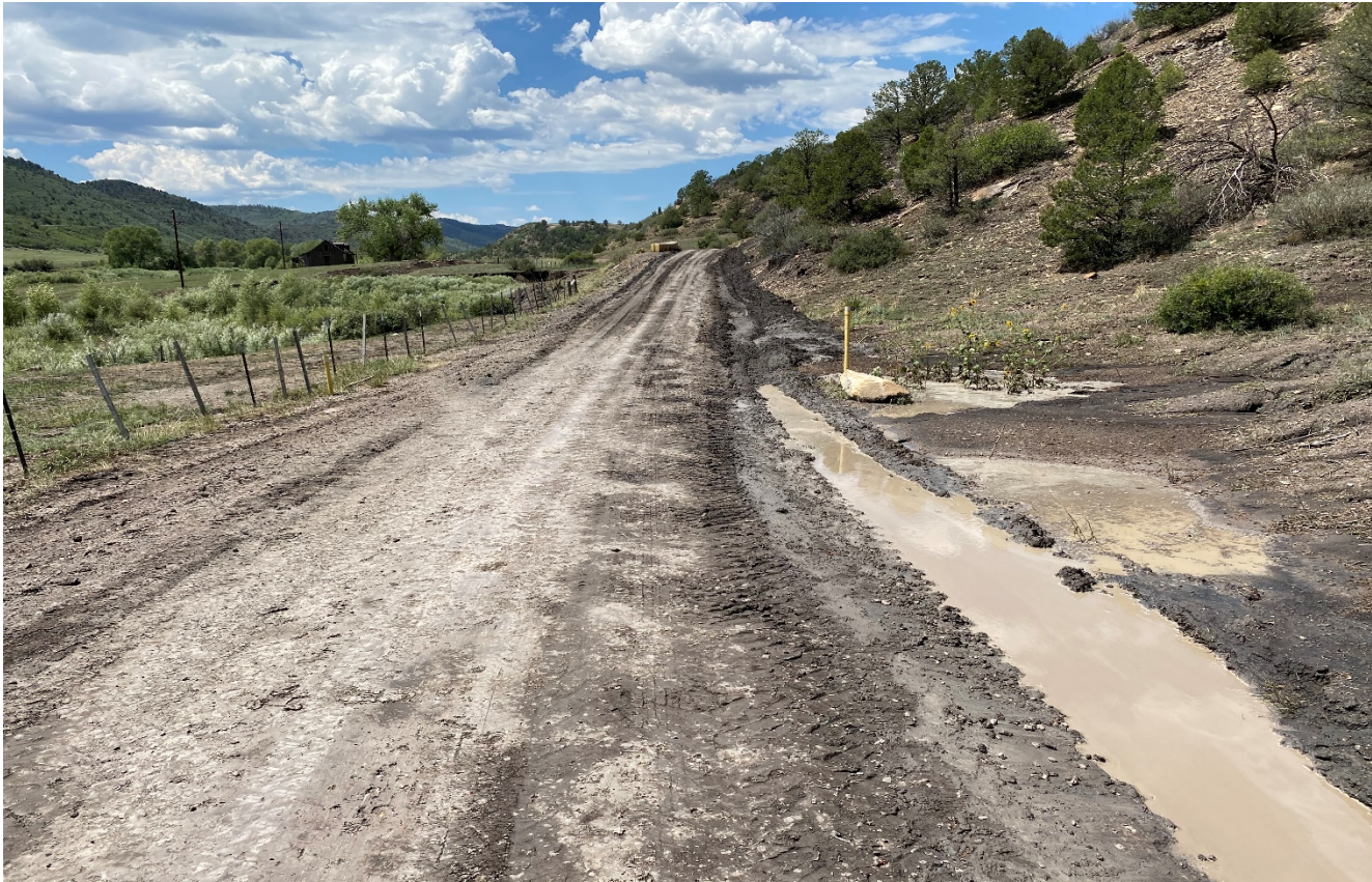
Photo 1. Facing southwest along the main road in the South Fork. Significant storm events have caused erosion along the road. Culverts are filled in with sediment and need to be cleaned out and maintained.
