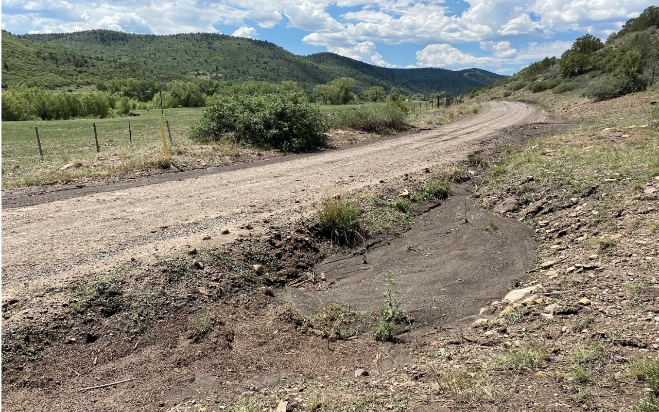
Photo 3. Further along the road are additional culverts filled in with sediment as shown in this photo.
