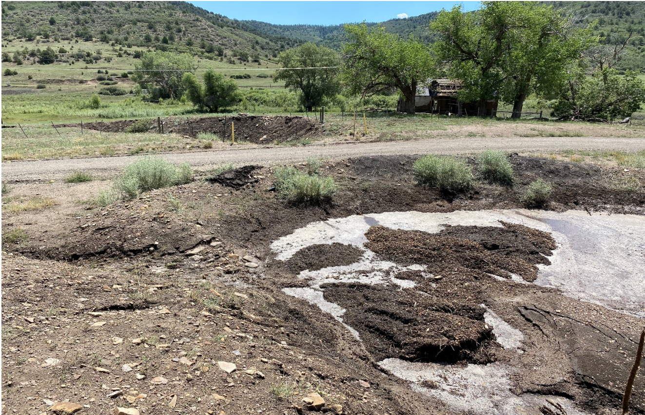
Photo 2. There is a culvert at this point along the road which is filled in with sediment causing water to not properly drain. The next storm event could cause erosion additional erosion and degradation of the road. The culvert needs to be cleaned out.
