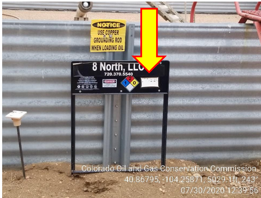
Photo 5 – 100 BBL Produced Water Tank missing Capacity
