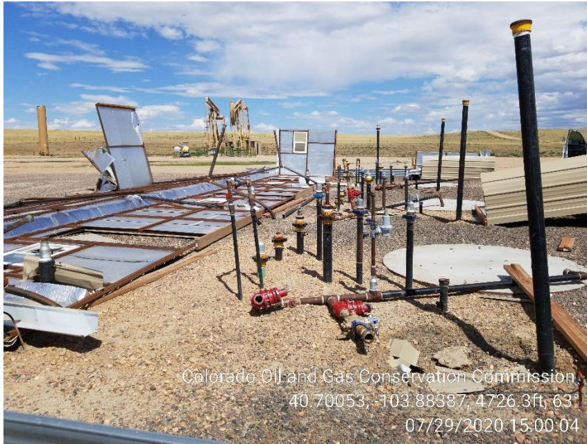
Photo 7 – Unmarked Risers, Debris, and unused pipes and fittings
