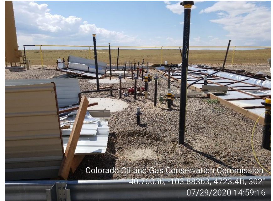
Photo 6 – Unmarked Risers inside berm
