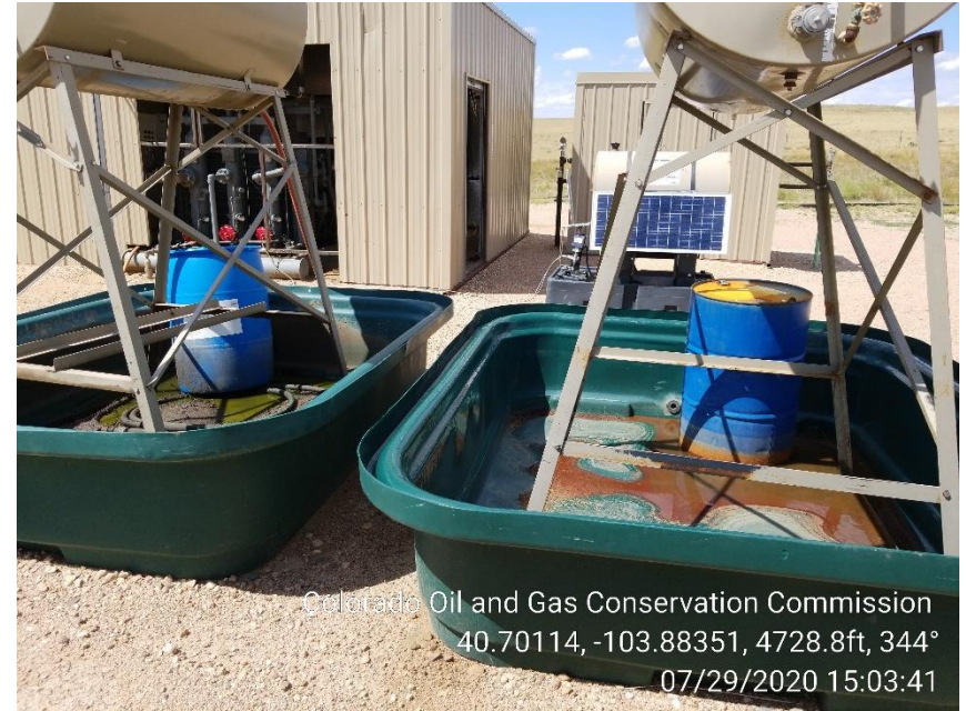
Photo 2 – Day Tanks at Compressor are missing Wildlife Netting
