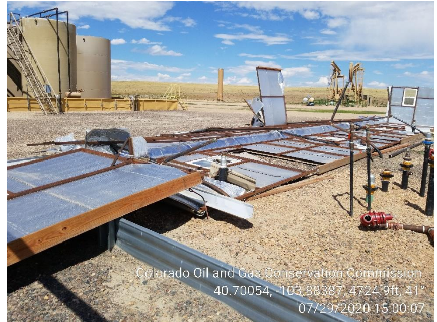
Photo 8 – Debris, Unused Equipment and Unmarked Risers
