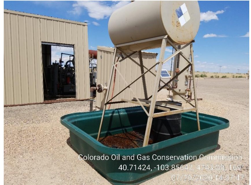
Photo 6 – Day Tank at Compressor missing Wildlife netting
