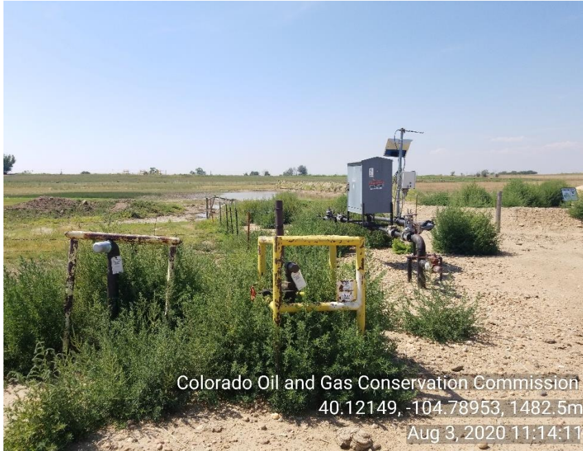
Photo 5 Risers have been tagged out. Weeds in and around equipment ( meter run)
