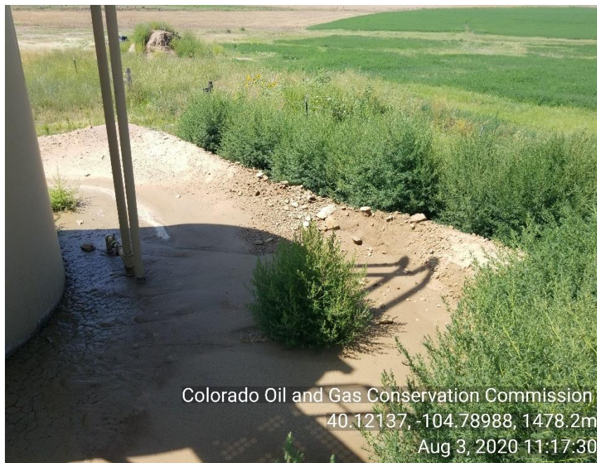
Photo 9 Berm appears to have been repaired but due to farmers sprinkler system containment has filled up and has blown out berm of containment around TNK BTRY. Weeds in and around TNK BTRY.
