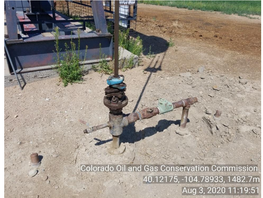
Photo 12 Appears well head leak has been addressed.
