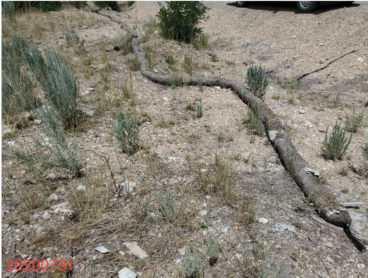
Photo 6: Photo taken from the east end of the Location. Photo shows straw wattles have not been installed or maintained in proper functioning condition.
