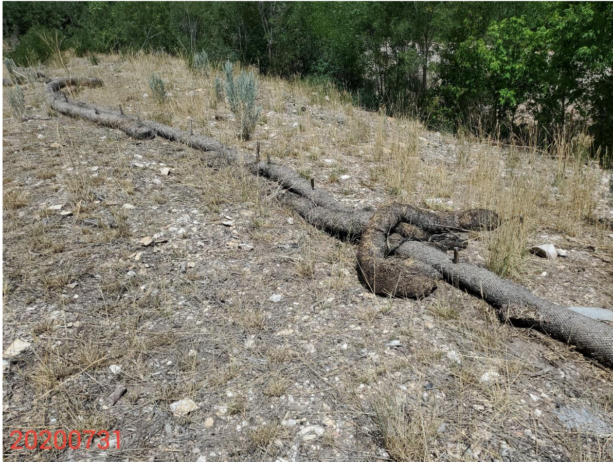
Photo 5: Photo taken from the east end of the Location. Photo shows straw wattles have not been installed or maintained in proper functioning condition.
