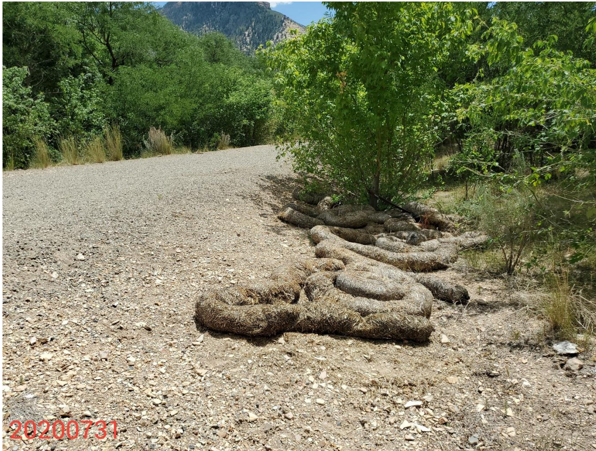
Photo 7: Photo taken from the ditch on the east end of the Location. Phot shows wattles within ditch; this is now considered debris.
