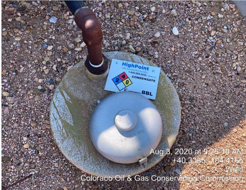
Photo #10 Missing capacity label
