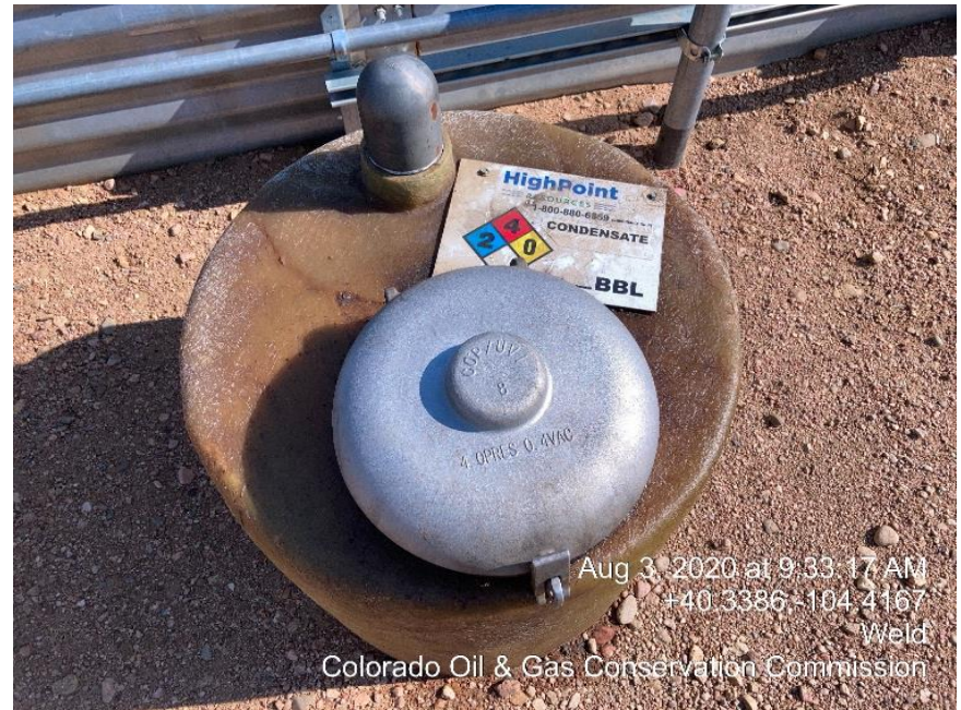
Photo #9 Missing capacity label
