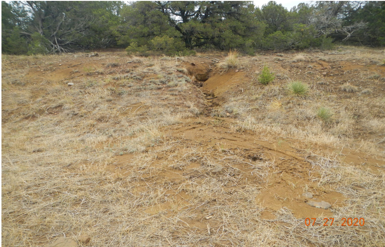
Photo 7. There is an erosion channel that has developed along the cut slope.
