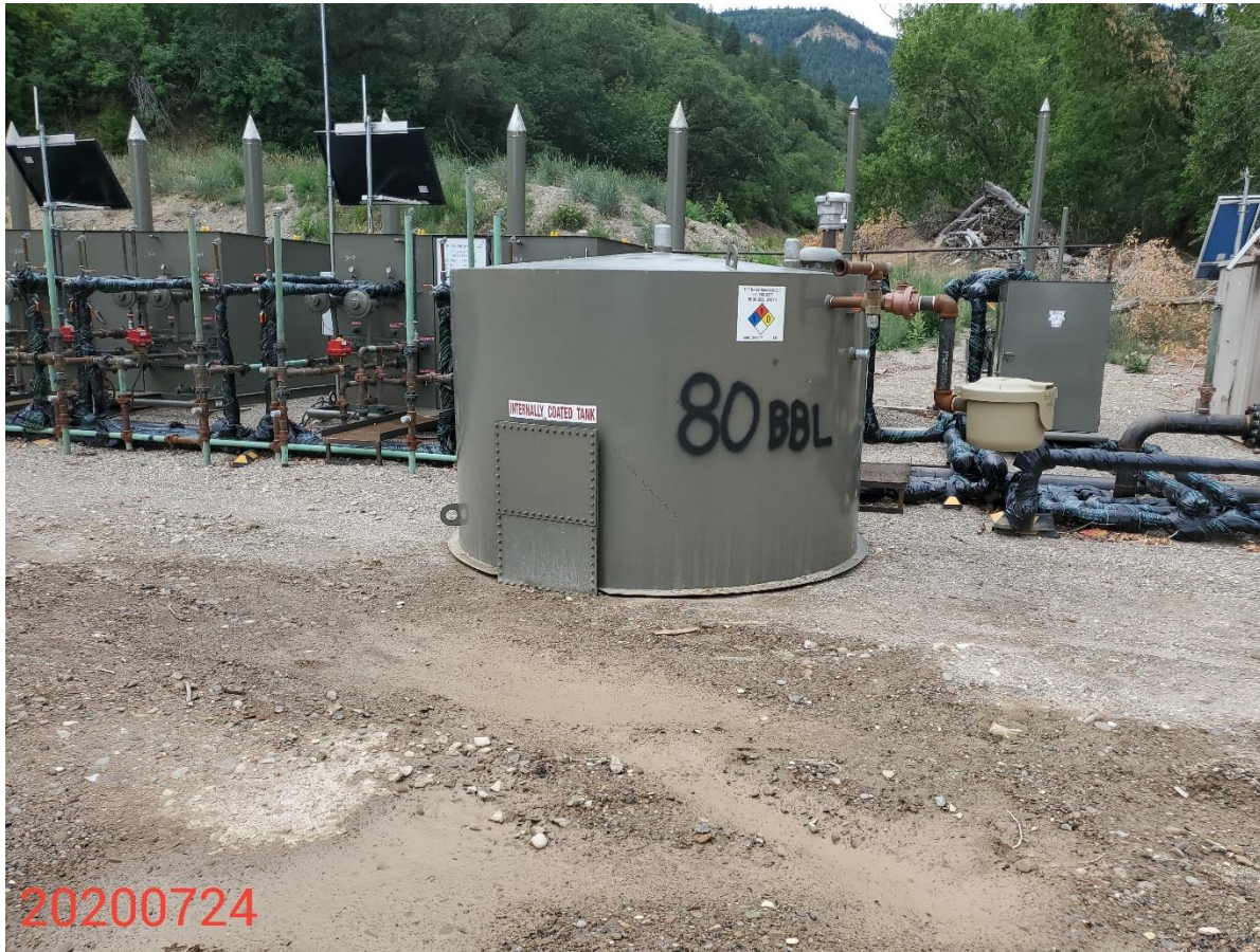
Photo 4: Photo taken from the south end of the Location, facing south. Photo shows 80 bbl produced water tank. Tank is not connected and appears to be unused equipment.
