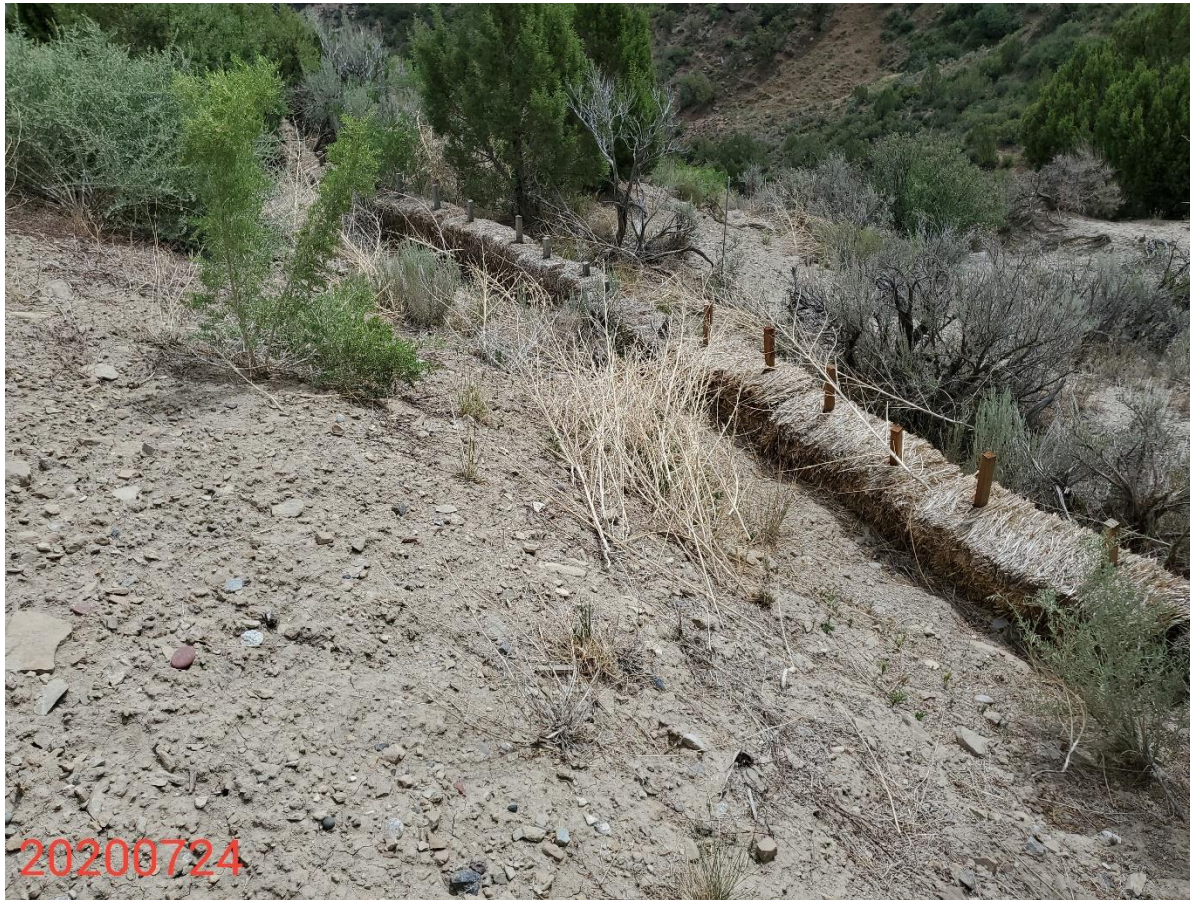
Photo 12: Photo taken from the southeast end of the Location. Photo shows hay bale BMPs. BMP appears to be in proper functioning condition.
