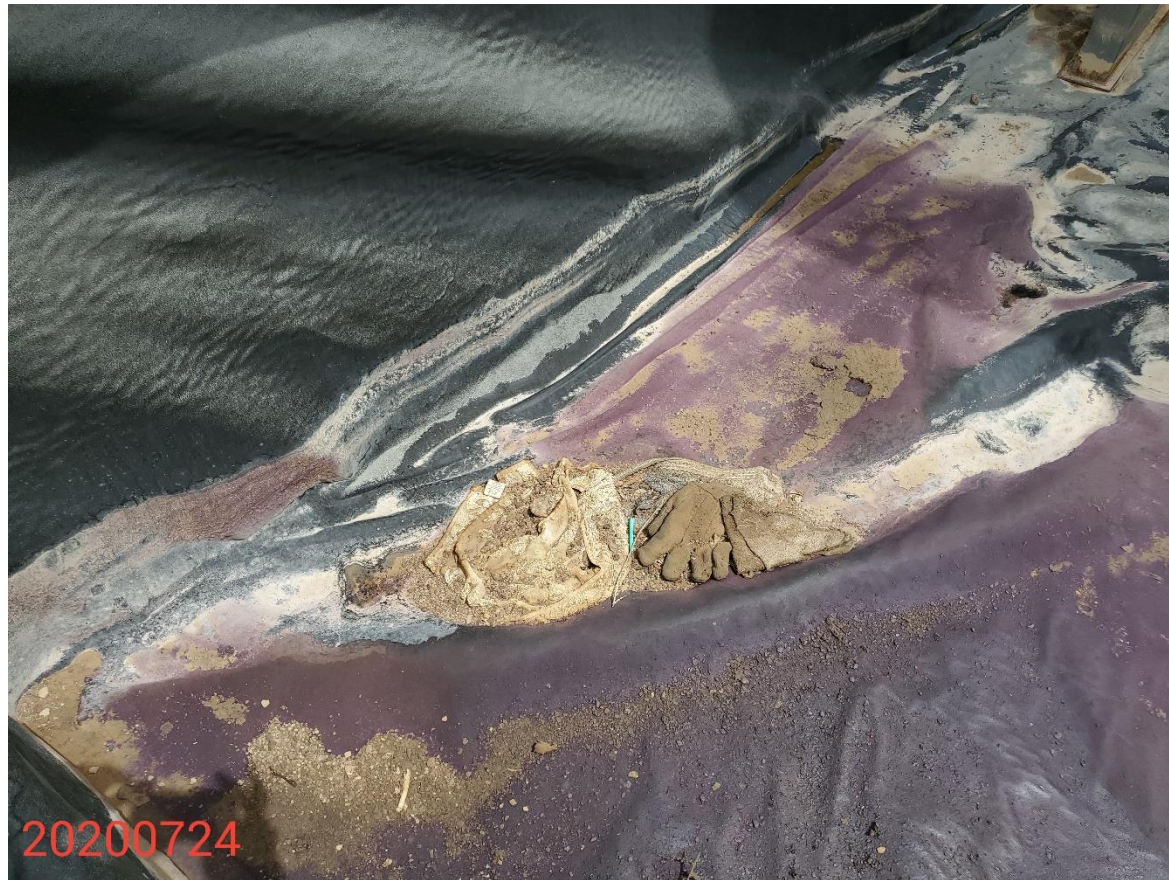
Photo 16: Photo taken from the containment berm at the tanks. Photo shows trash debris stored within containment.
