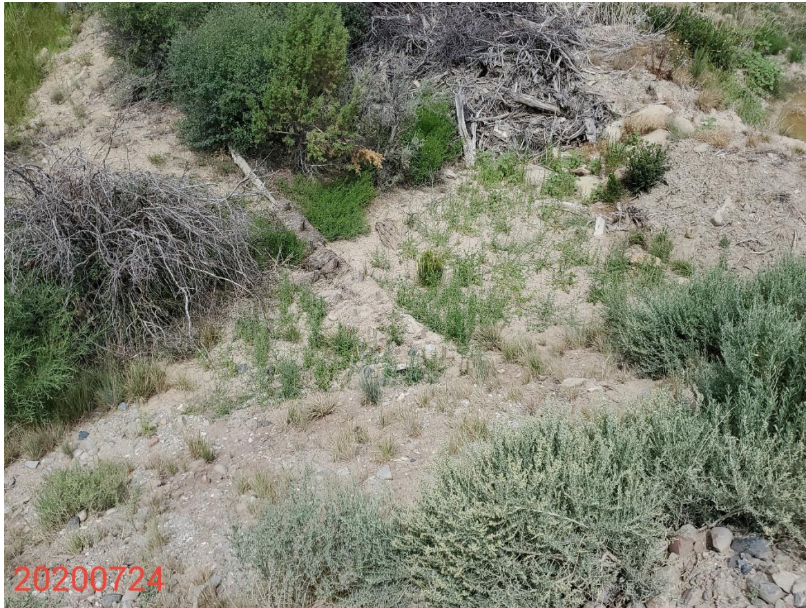
Photo 14: Photo taken from the sediment trap to the south of the Location. Photo shows hay bale BMP installed at outlet of trap has filled with sediment, and is no longer in proper functioning condition.
