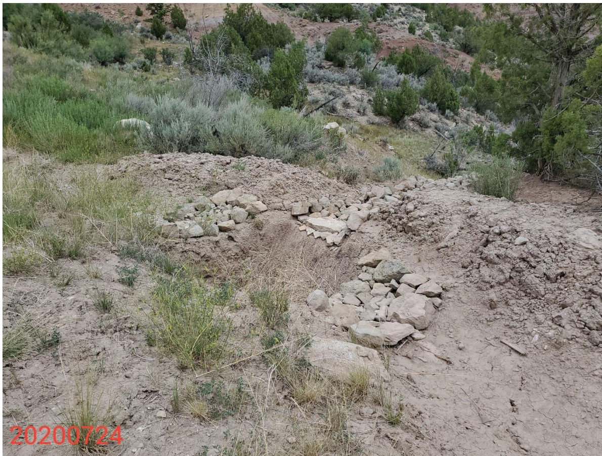
Photo 5: Photo taken from the north end of the Location, facing north. Photo shows sediment trap. BMP appears to be in proper functioning condition.
