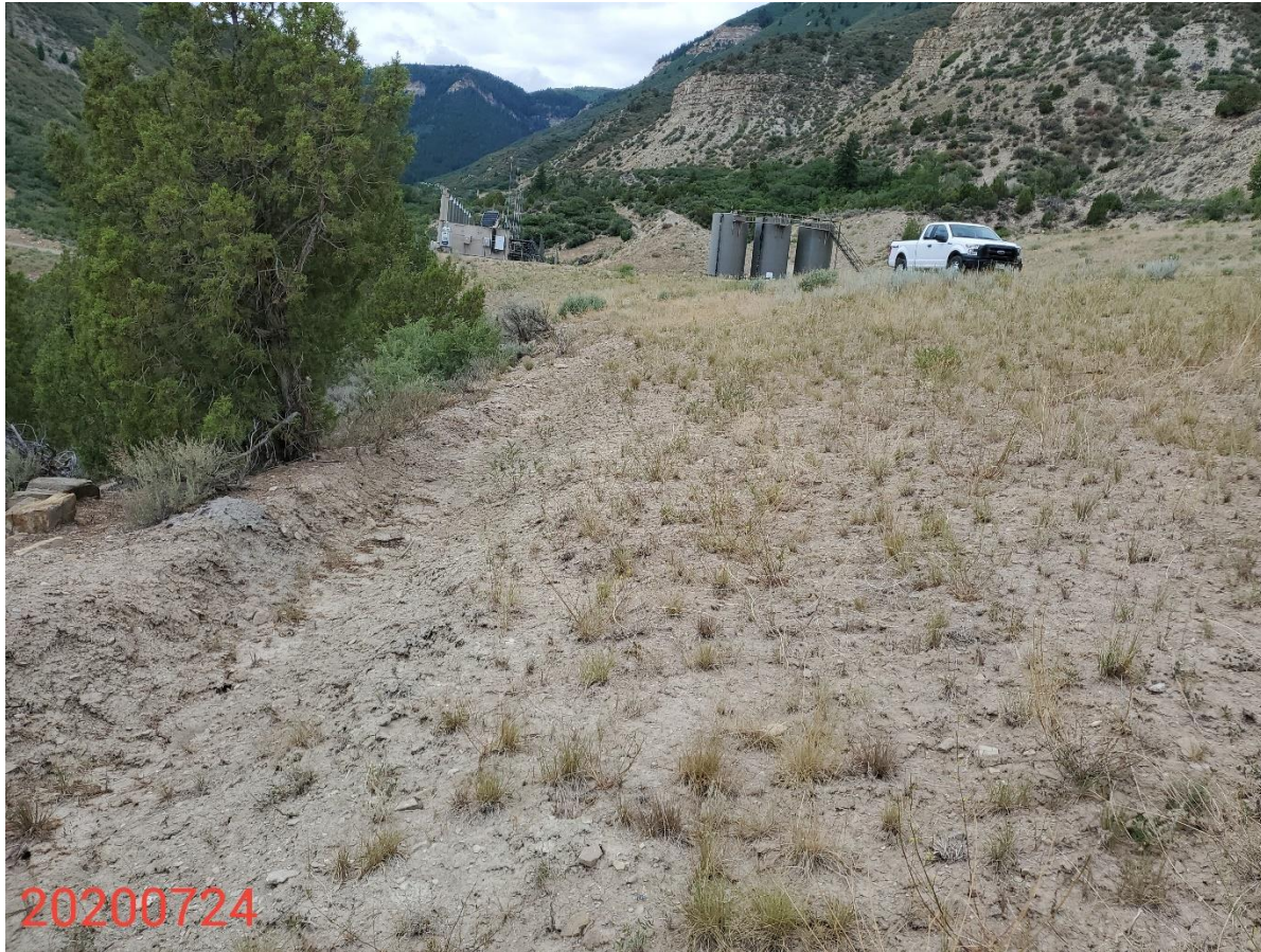
Photo 6: Photo taken from the northeast end of the Location, facing south. Photo shows stormwater diversion ditch along the eastern perimeter of the Location.
