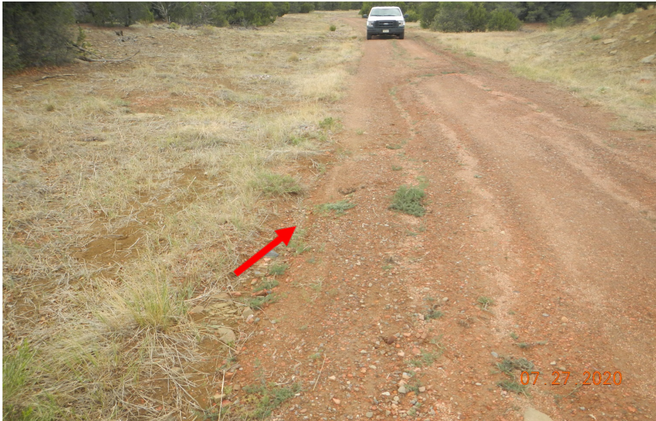
Photo 2. There is signs of stormwater flowing down the road causing erosion.
