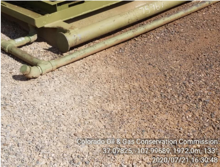
PHOTO 3: AREA OF IMPACTED SOIL NEAR FRONT OF COMPRESSOR. Conduct maintenance on equipment, cleanup stained material and review self inspection processes. CA DATE 10-21-20.
