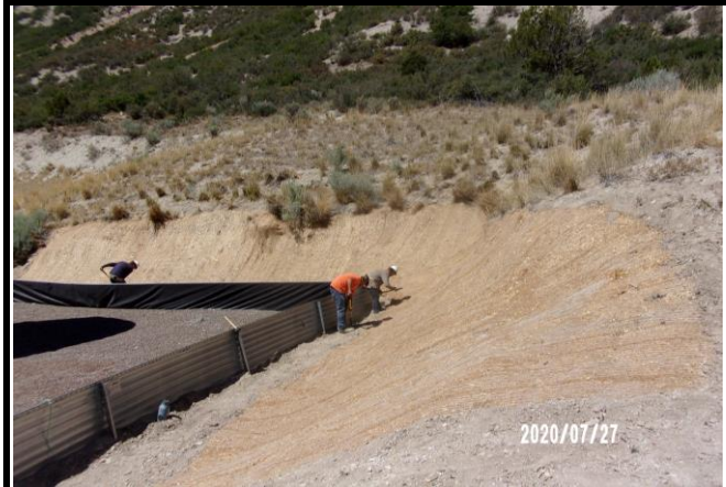
Curlex Installation on the C.C. 632-13-22
