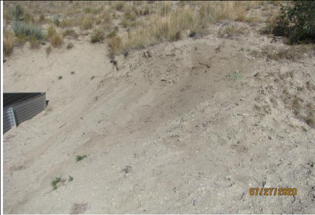
Fissure Repair on the C.C. 632-13-22
