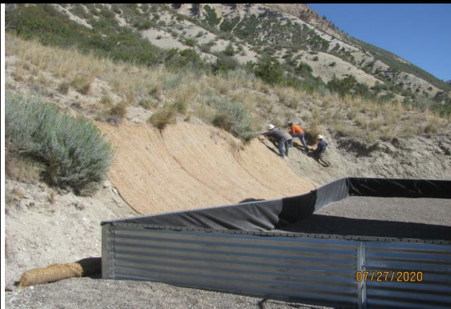
Curlex Installation on the C.C. 632-13-22
