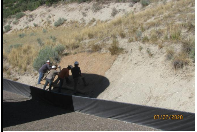
Curlex Installation on the C.C. 632-13-22
