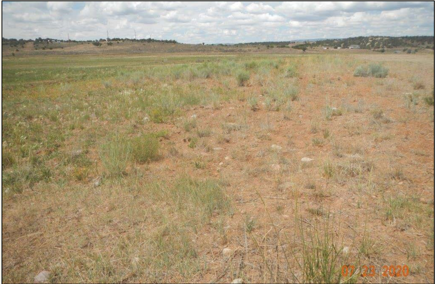
Photo 2. View of the southern fill slope from the southeastern corner facing westward. Revegetation is progressing with crested wheatgrass, western wheatgrass, and sand dropseed.
