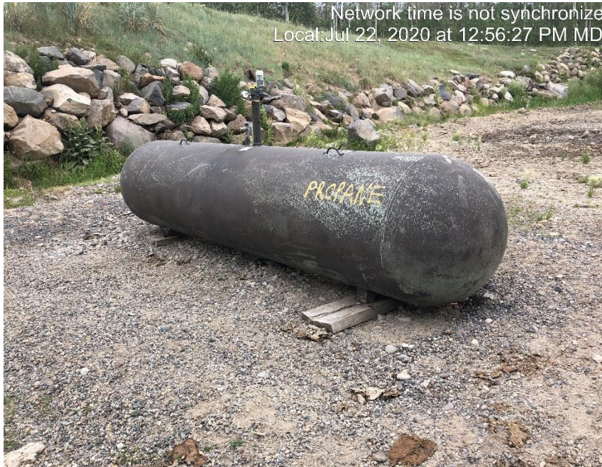
Photo #1584 Tank label propane missing NFPA label.
