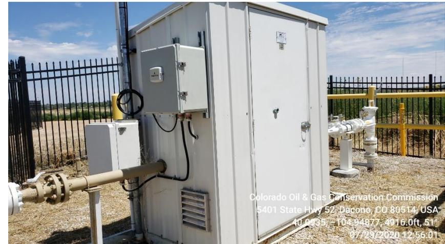
**Photo 7 Unused Gas Meter Run appears to be not connected to production lines**
