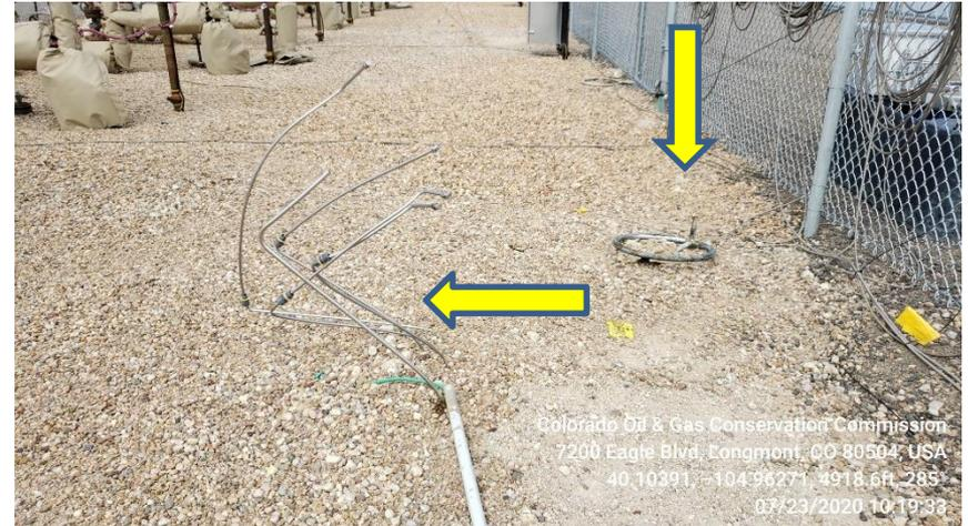
**Photo 6 unused stainless steel lines ,valve handle**
