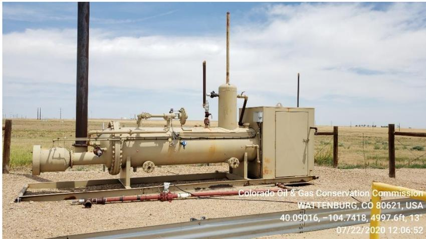
**Photo 7 Unused Horizontal Heated Separator**
