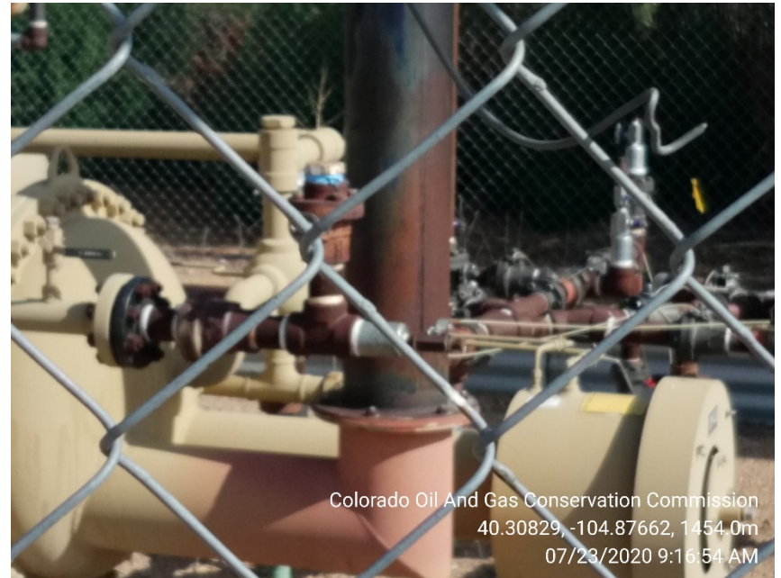
Disconnected separator gas sales line
