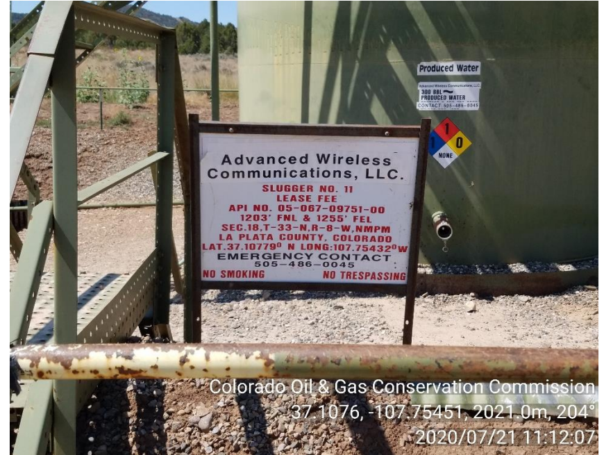
PHOTO 2: WELL SIGN/ 911 NOT LISTED AS EMERGENCY CALL NUMBER ON BATTERY SIGN. INSTALL SIGN TO COMPLY WITH RULE 210.b. CA DATE 10-21-20.
