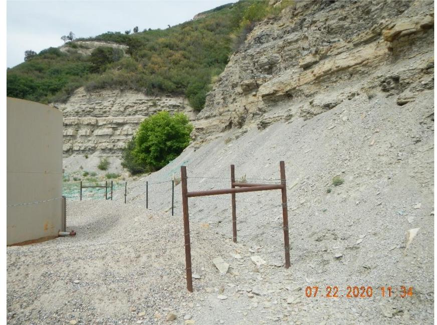
**Sediment around unstable cut slope continues to build up.**
