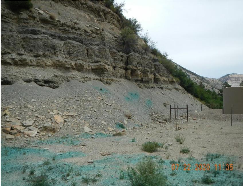
**Sediment around unstable cut slope continues to build up.**
