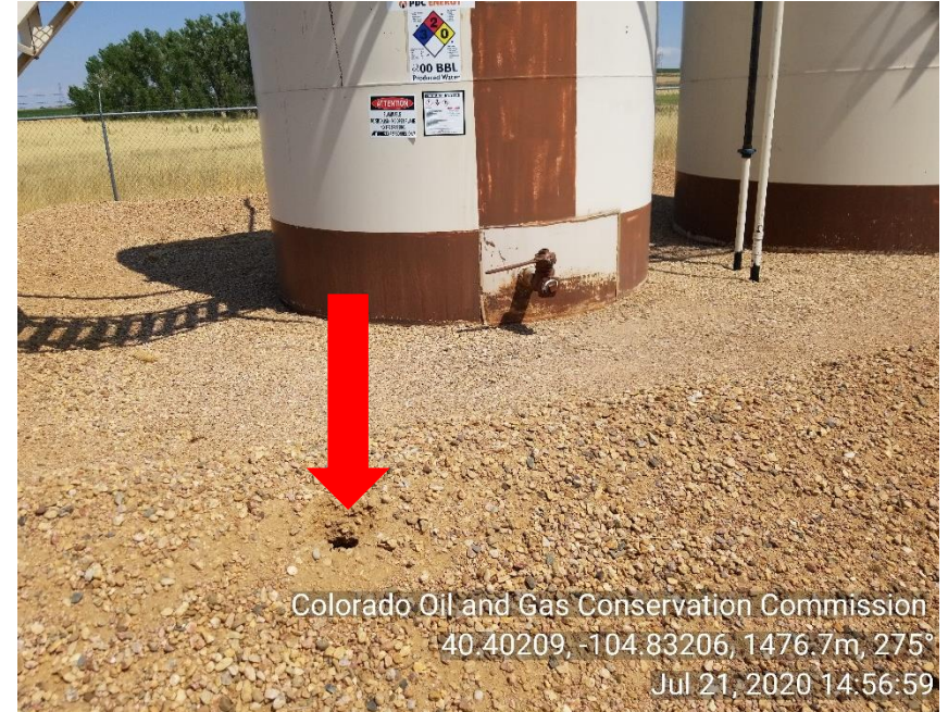
Photo 8: Hole in berm
