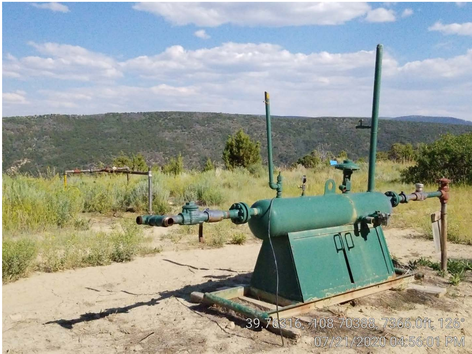
Photo 3. Separator & riser.
