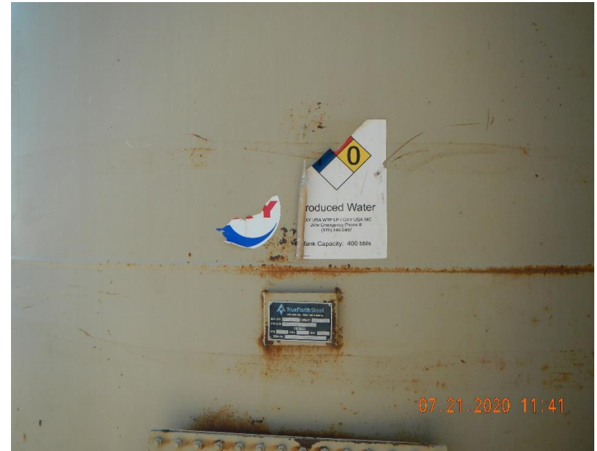
Tank stickers are damaged.
