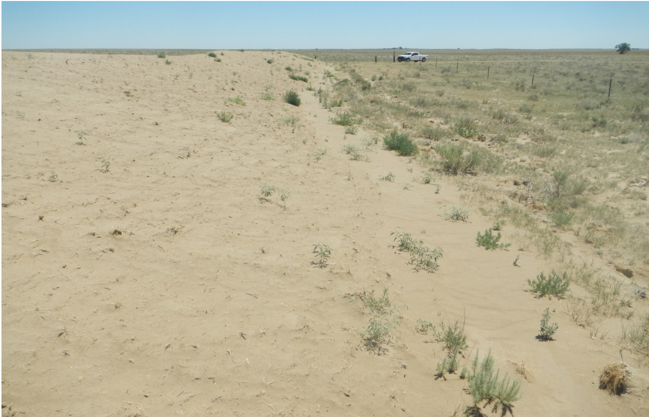
Photo 4. Facing south at backside of the topsoil pile. There is wind erosion occurring of the sandy soils. The soils are not stabilized and there are insufficient BMP's.
