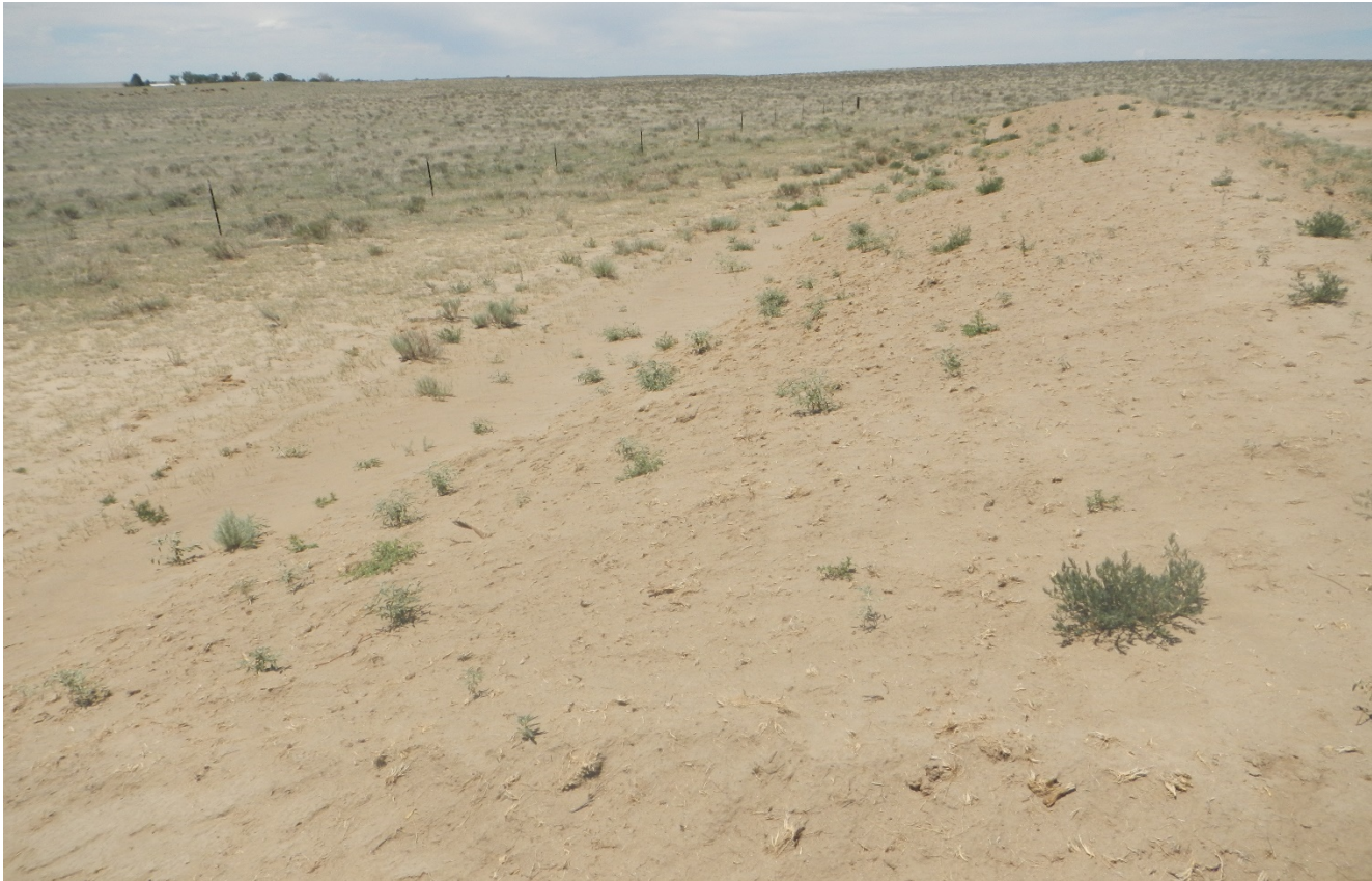
Photo 8. Facing toward the backside of the soil pile at eastside of the location. There is wind erosion occurring of the sandy soils. The soils are not stabilized and there are insufficient BMP's.
