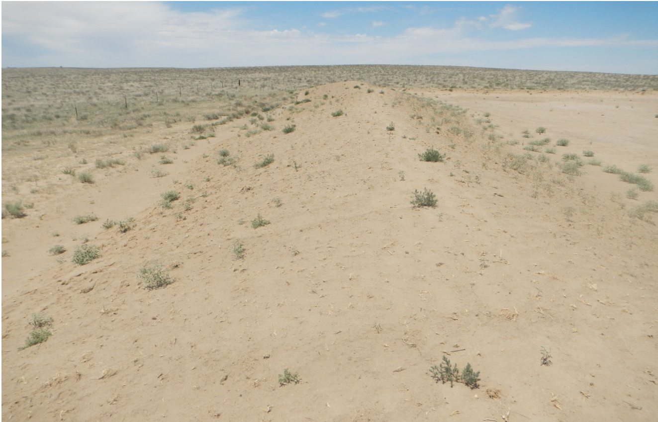
Photo 3. Facing north on topsoil pile. The soil is not stabilized and there are signs of erosion.
