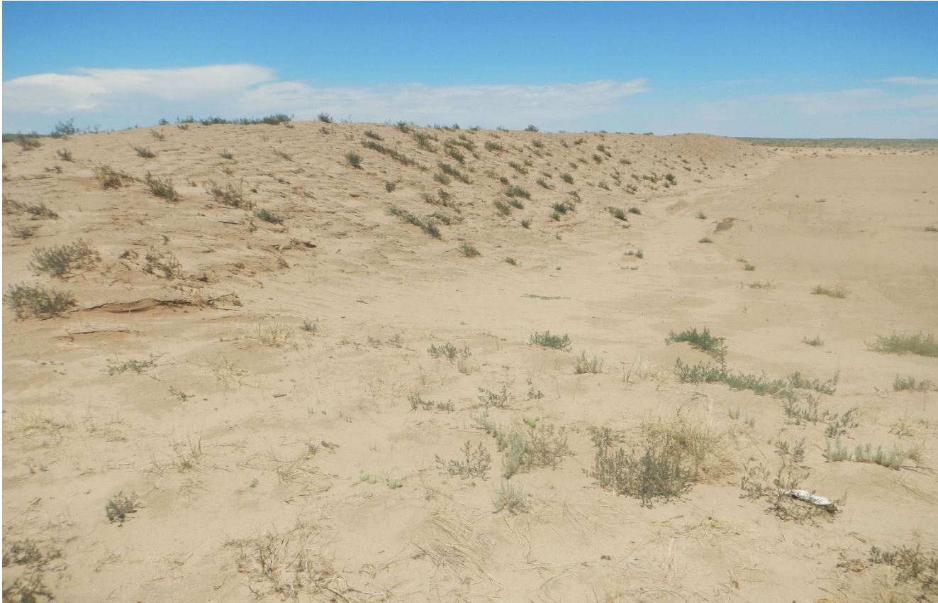
Photo 3. Facing toward the topsoil pile. The soil is not stabilized and there are signs of erosion.
