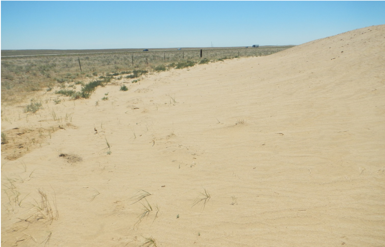
Photo 9. The sandy soils have eroded offsite and there is no perimeter erosion controls.
