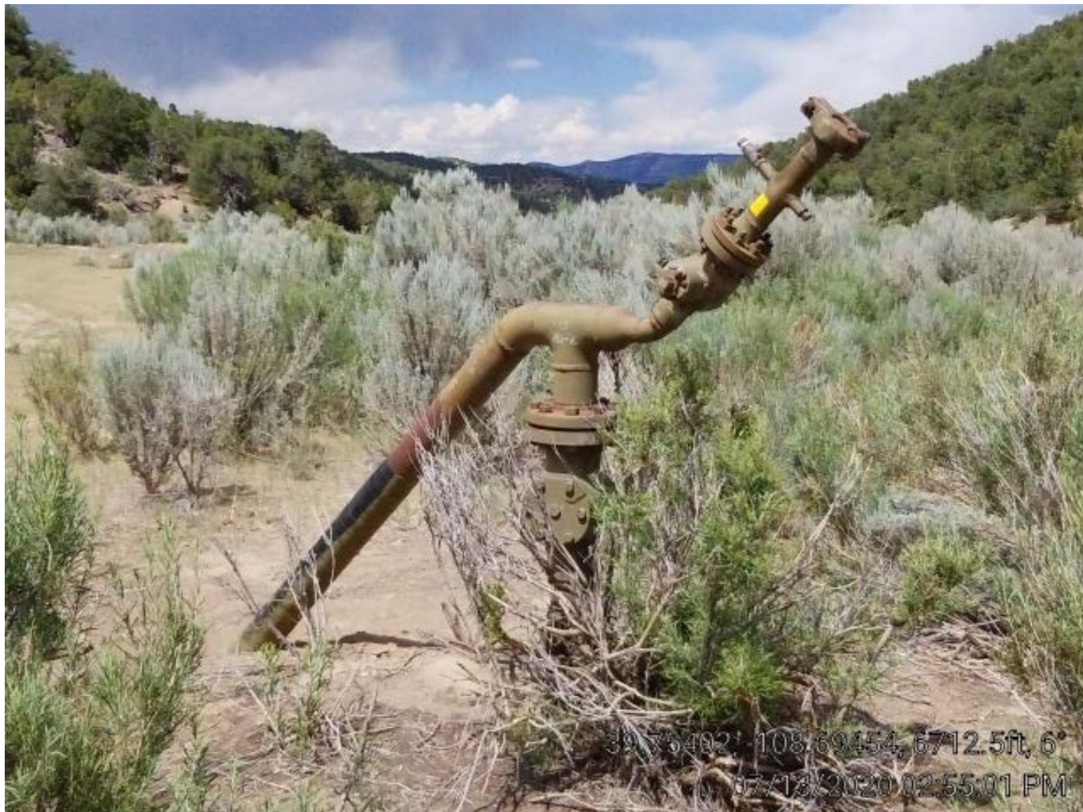
Photo 4. Flow line riser.
