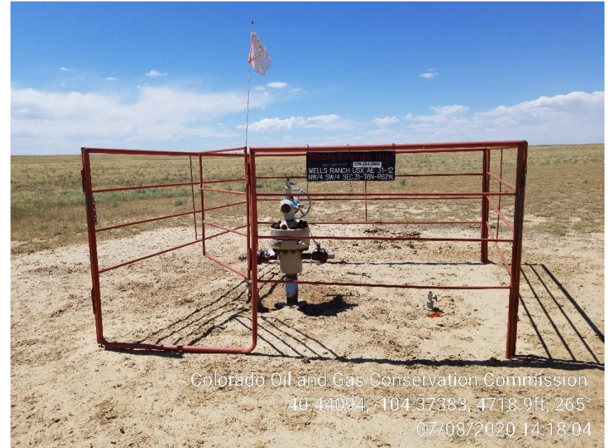
Photo 2 – Wellhead Variance Tag not installed
