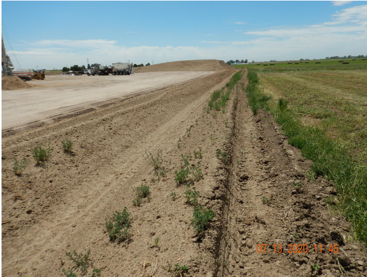
Photo 1. Photo taken from the northwestern perimeter of location, facing South. Photo illustrates a ditch BMP which has been installed around the entire perimeter of the location.
