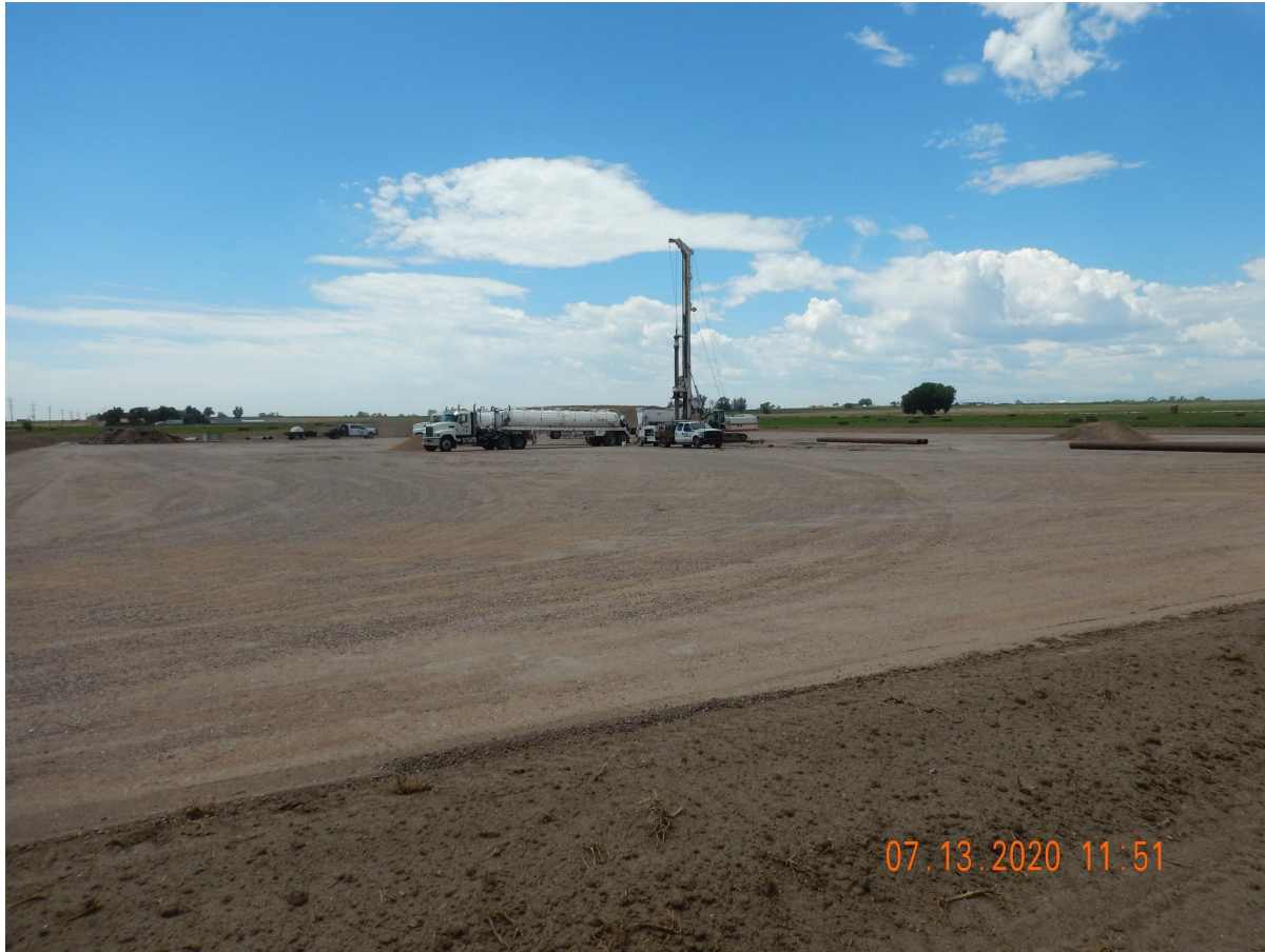
Photo 8. Photo taken from the northern perimeter of location, facing South. Photo illustrates the Operator is setting conductors.
