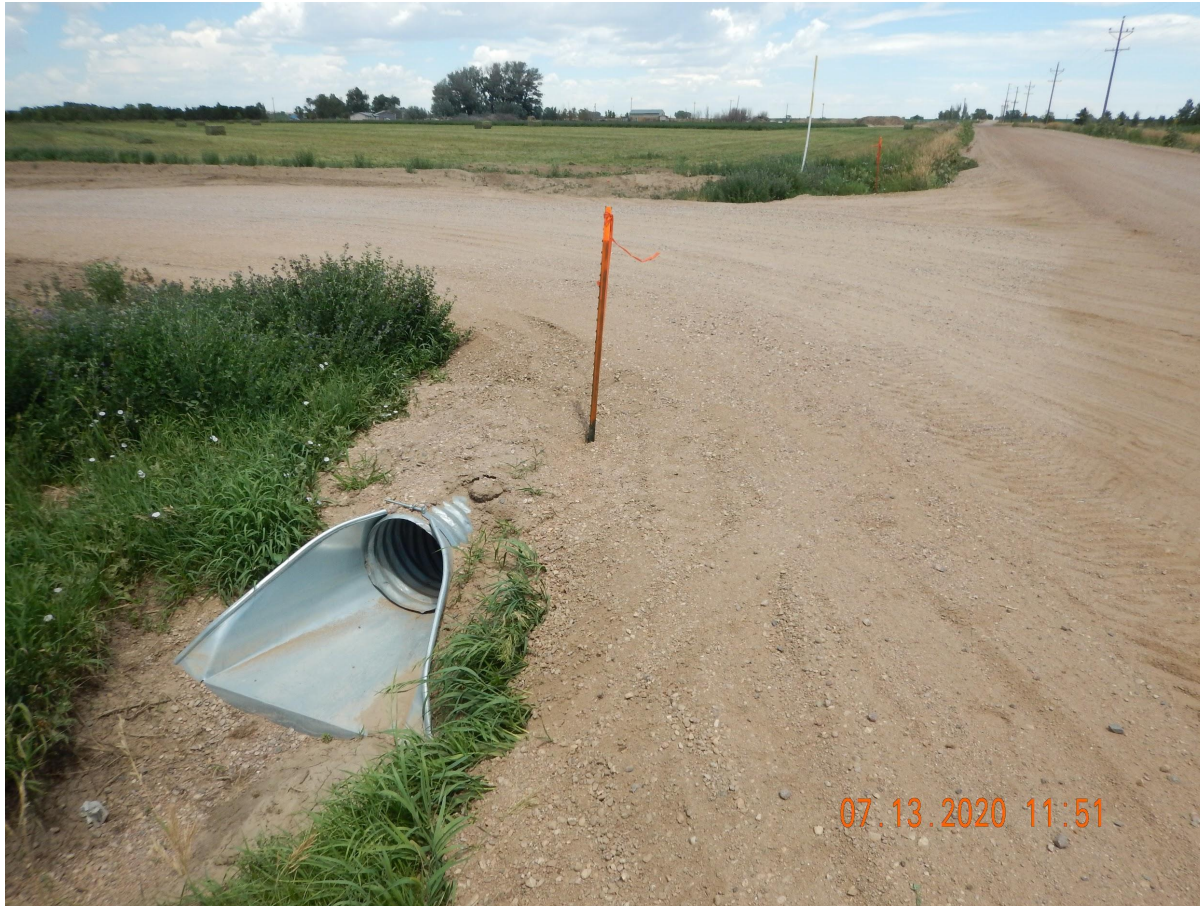
Photo 6. Photo taken from the entrance of location, facing North. Photo illustrates the Operator has installed a culvert in conjunction with the roadside ditch.
