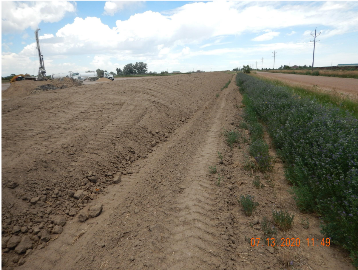
Photo 5. Photo taken from the southeastern perimeter of location, facing North. Photo illustrates the eastern topsoil stockpile which has been temporarily stabilized.
