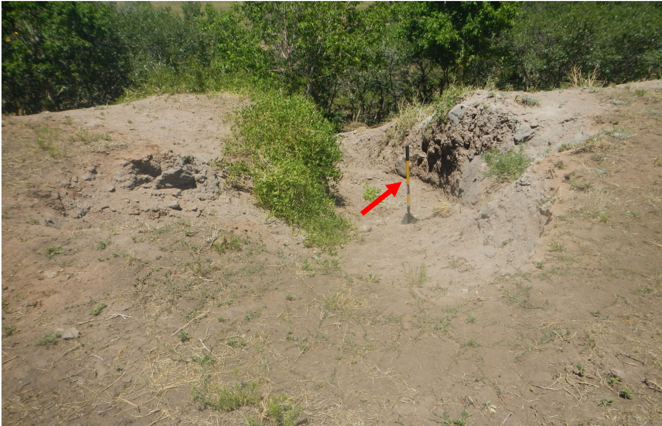
Photo 13. There is a deep gully erosion of the northeast fill slope. Red arrow points to 4.5 ft. shovel to show side of erosion.
