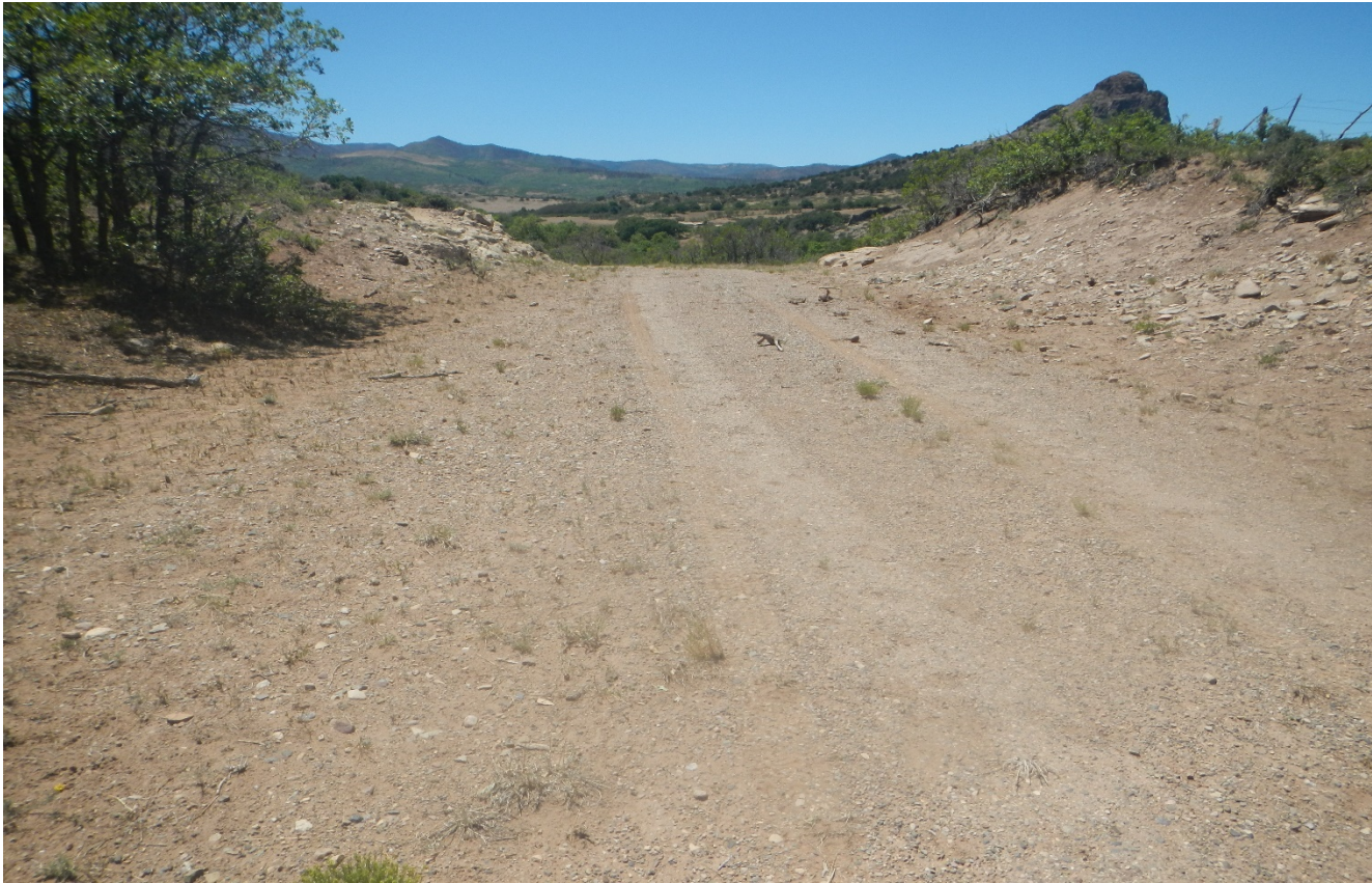
Photo 4. Facing south along the access road. Access road has not been recontoured and reclaimed.
