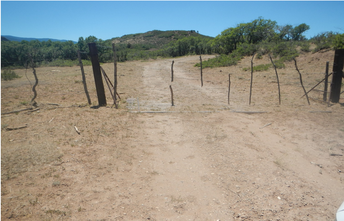
Photo 3. Facing south along the access road. The cattle guard remains and is filled in with sediment.
