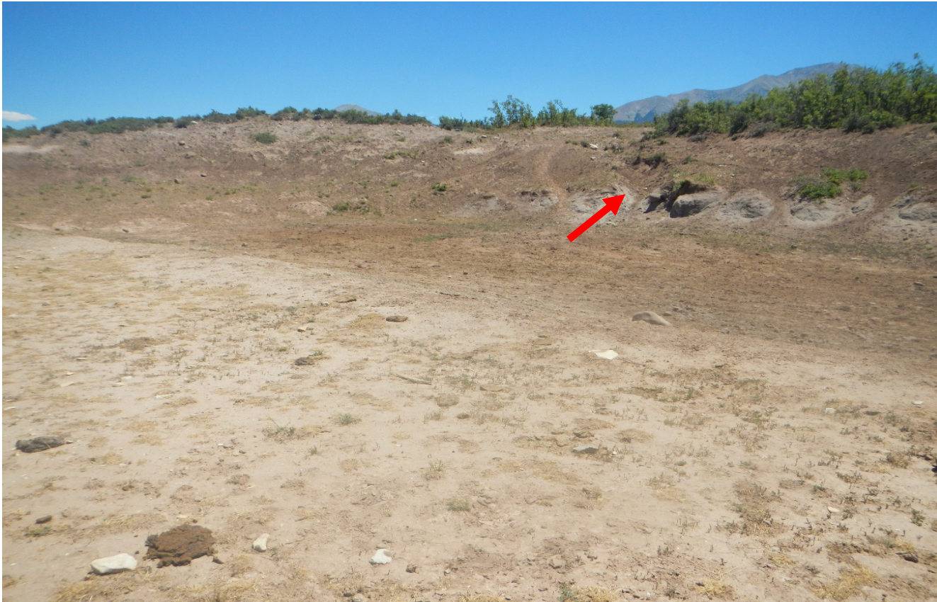
Photo 9. Facing southeast toward the cut slope of the location which is approximately 30 ft. height. Red arrow points to an erosion channel at the cut slope.
