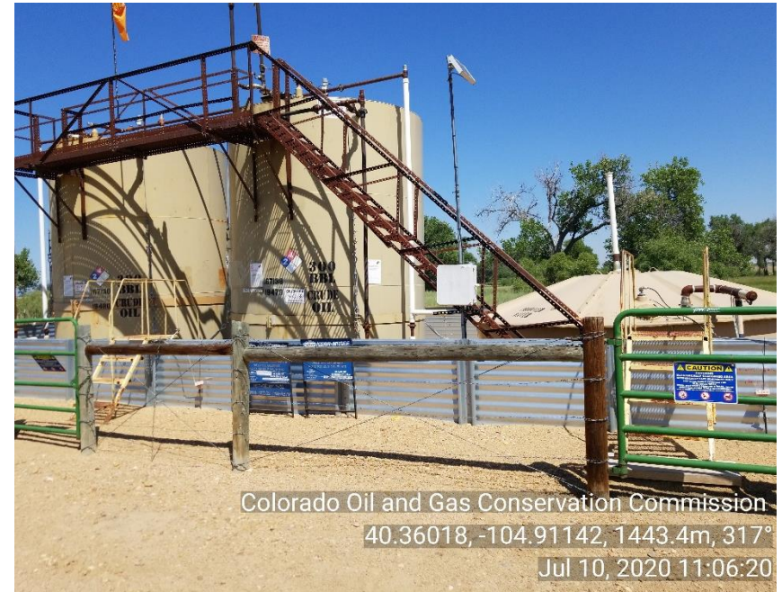
Photo 4: Tank Battery
