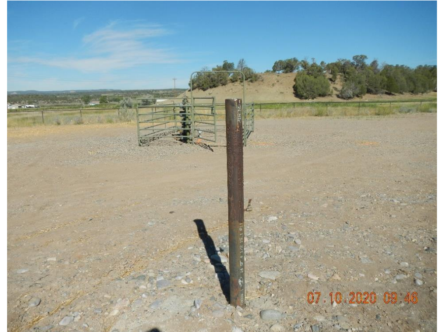
PA marker for 067-08022 and State CB #1 well head with stock panel enclosure.
