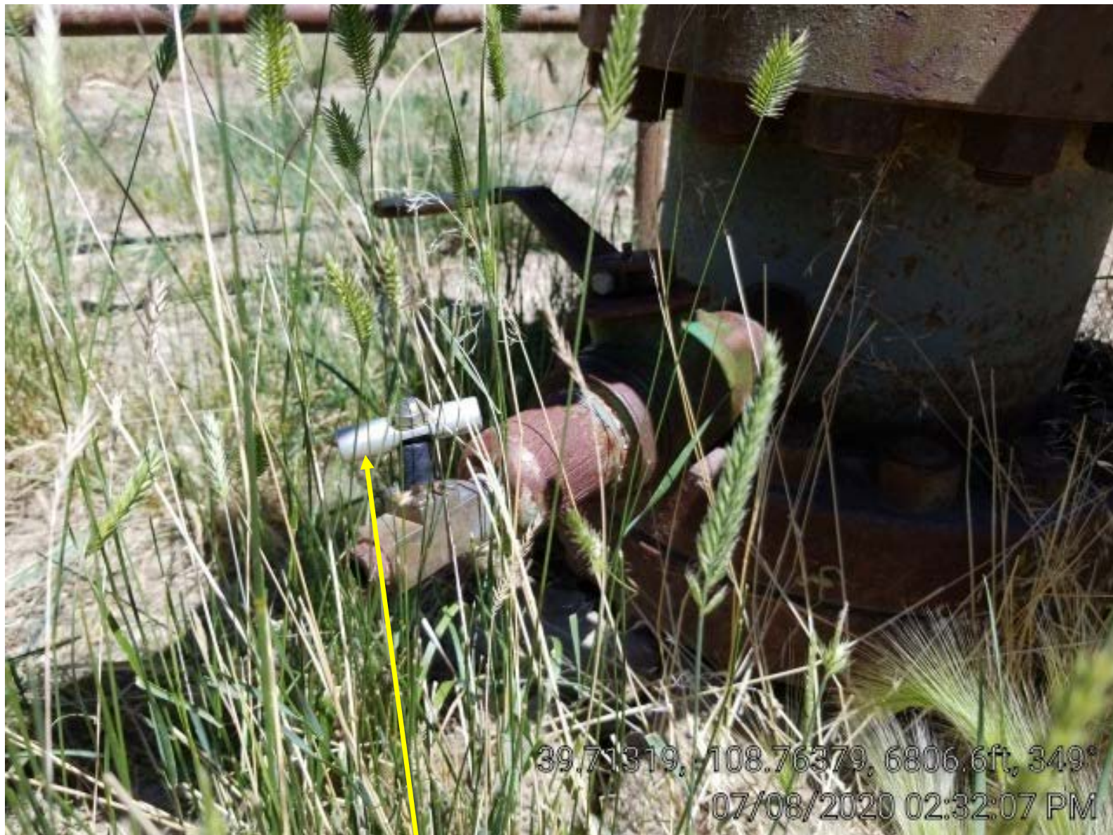
Photo 4. Open bradenhead valve.
