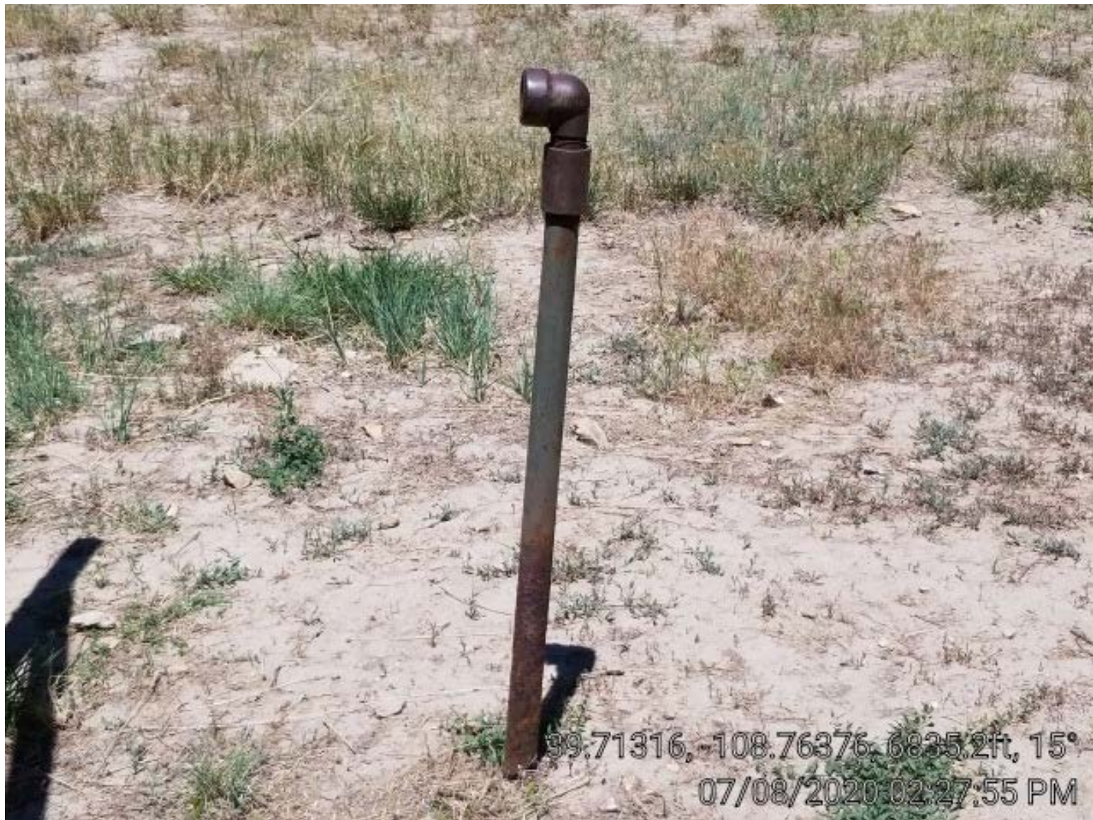
Photo 5. Uncapped riser next to well.
