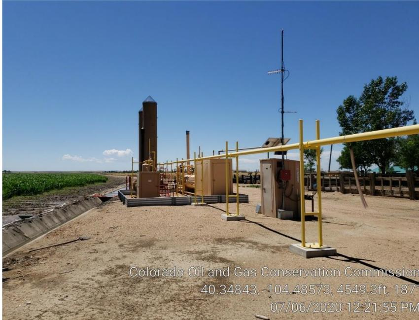
**Photo #3 Separators, ECD's & meter run**
