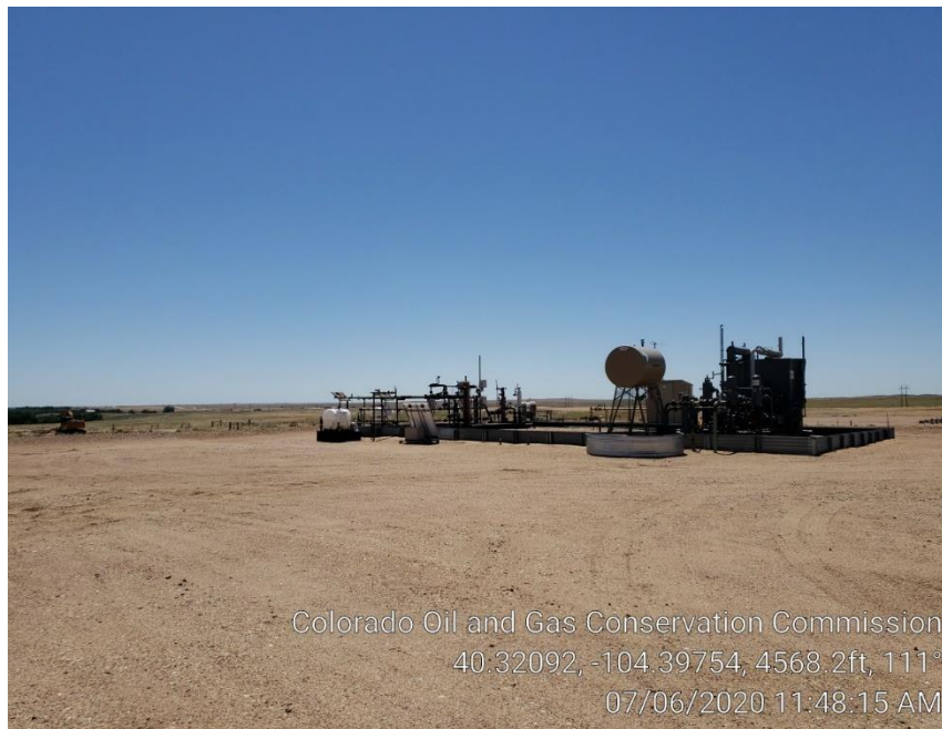
Photo #3 Compressor, gas lift & Meter run
