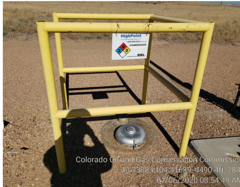
Photo #13 Missing capacity label
