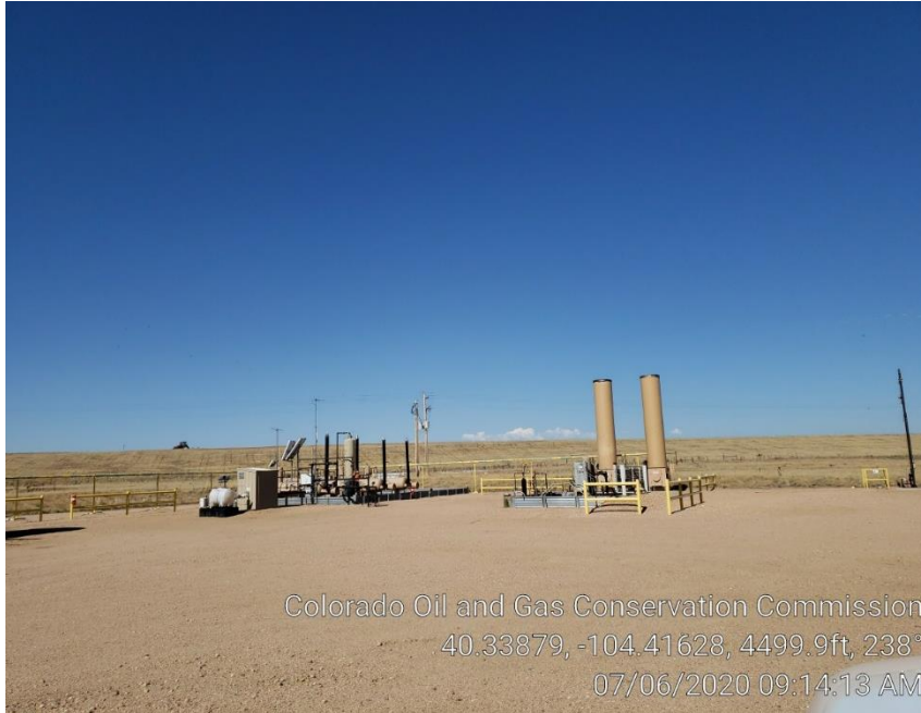
Photo #3 Separators, ECDs, VRU & Flare
