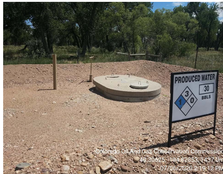
Produced water vault anchoring and berm
