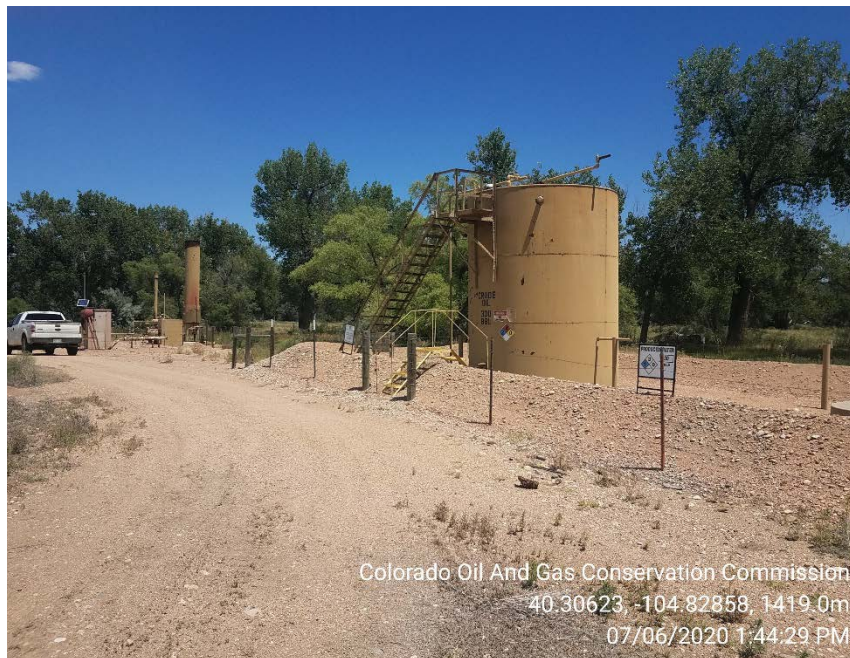
Tank battery and berm
