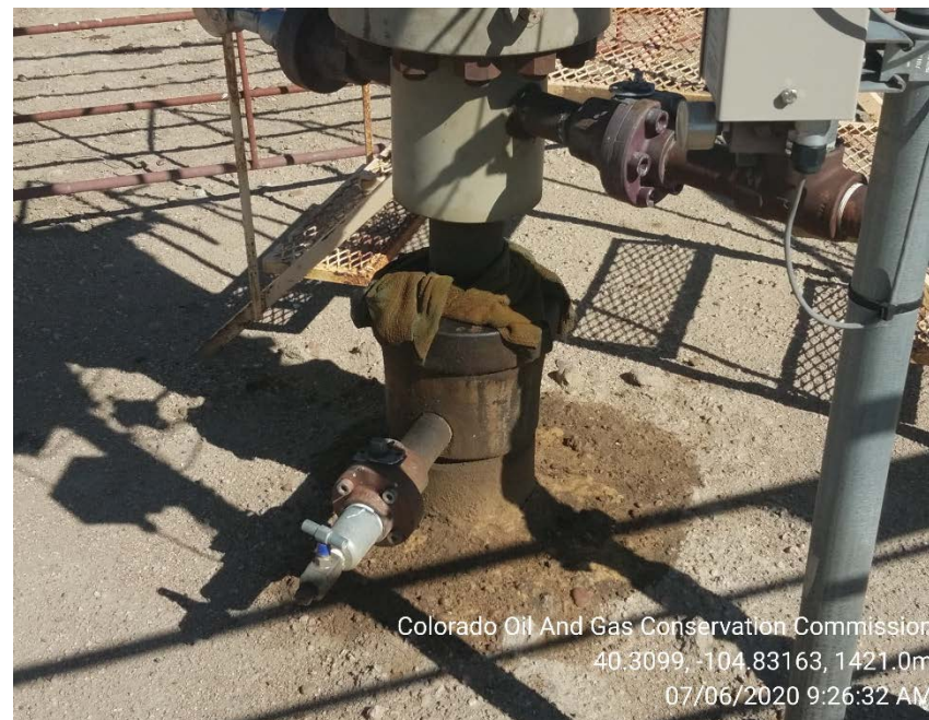
Bradenhead packing and stained soil
